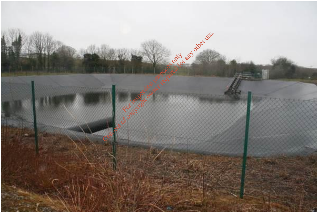
Figure 2.10 Fire water retention pond
