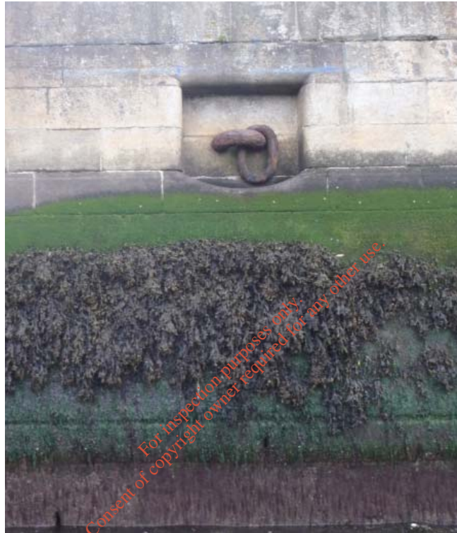
Plate 4.1 Existing Mooring Ring on North Wall Quay Extension
