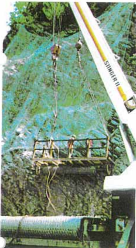
■ USA - Tennessee Erection of netting by means of a crane, along Interstate 40.
