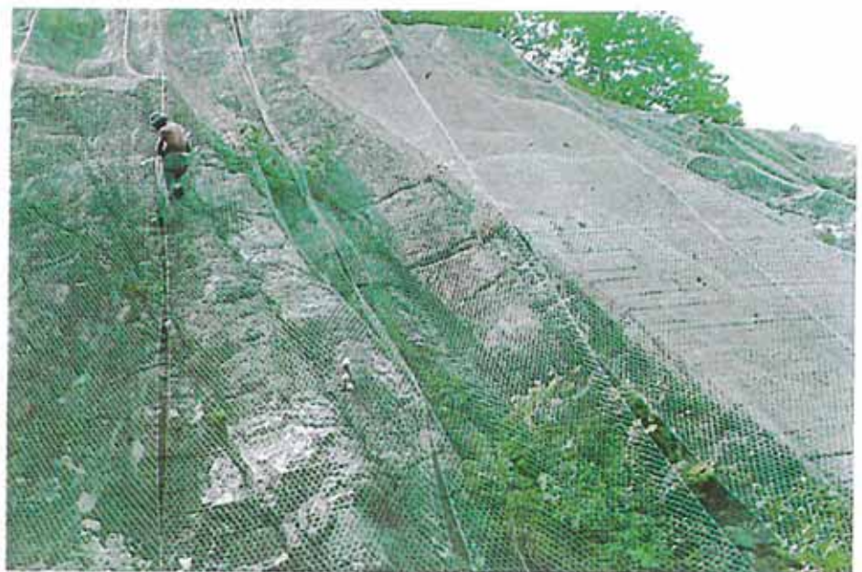
■ ITALY Lacing the netting.
