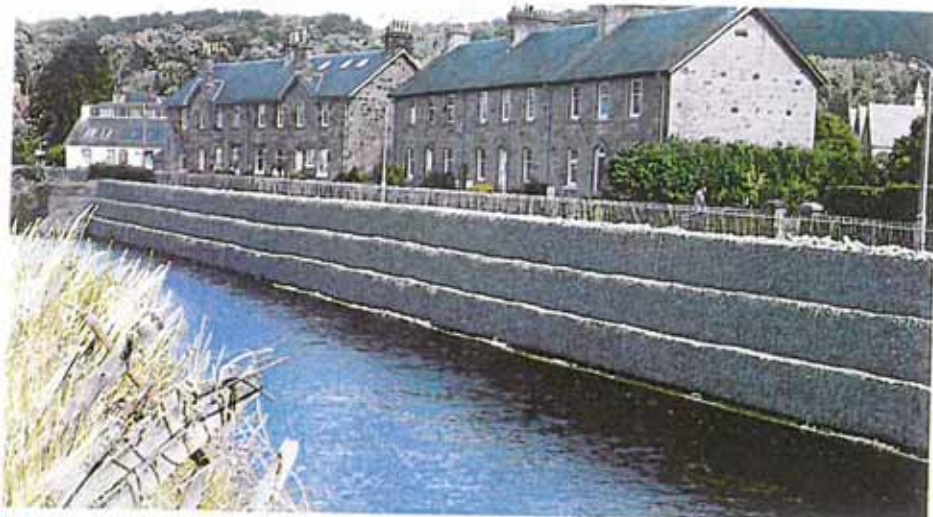
■ SCOTLAND Gabion wall flood protection at Bridge of Allan.
