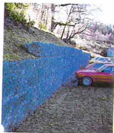
■ SCOTLAND Gabion retaining wall at Dunkeld House Hotel, Perthshire.
