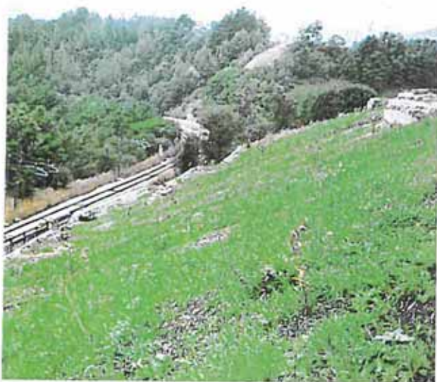
Italy - Trentino-Alto Adige Protection with MacMat-R® of slope overlooking a railway in Brunico-Bolzano, near Perca (BZ).
