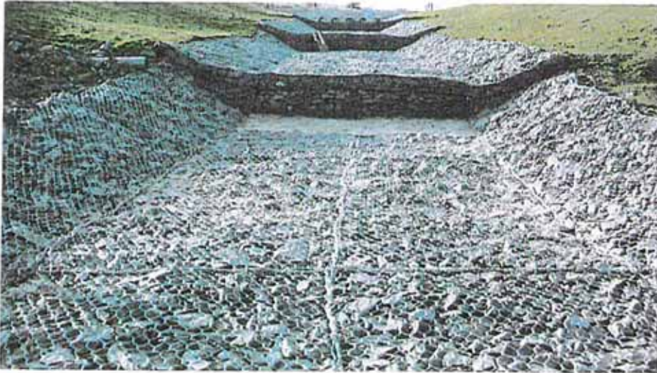
■ SCOTLAND - Dumfries & Galloway Reno® mattress spillway lining and drop structures, Torbeckhill Reservoir.
