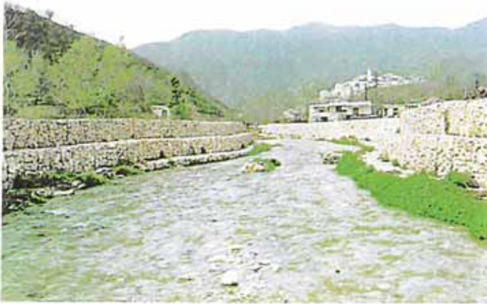
■ ITALY - Campania Longitudinal walls on River Lete.
