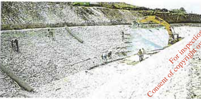
■ Reno® mattresses filling and closing operation.
