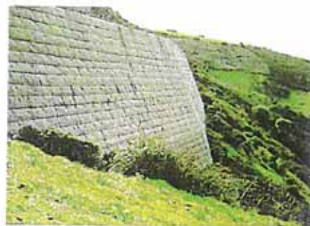
■ ITALY - Sardegna Retaining works carried out with Green Terramesh® units along the road Bitti-Lula which connects the SS131 to the SS389.
