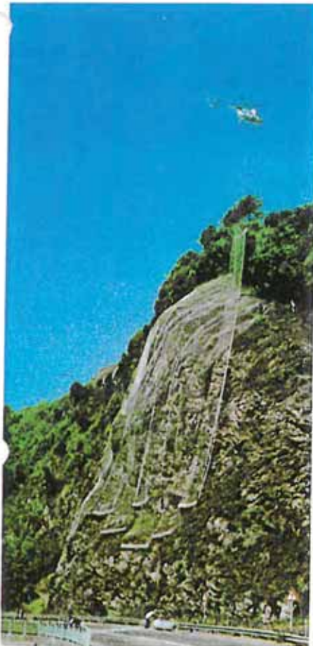
■ ITALY - Liguria Erection of netting by means of a helicopter, near Arenzano.
