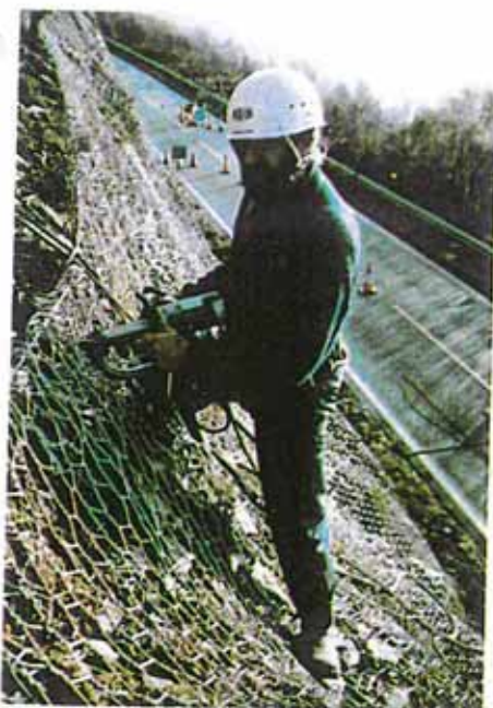
■ SCOTLAND Rock-netting installation, A835 South Ullapool.
