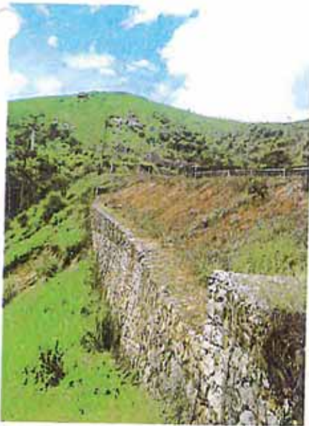
Example of differential settlement without fracture
