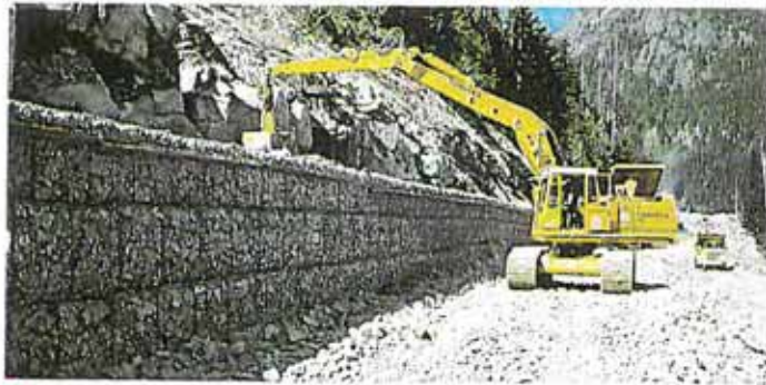
■ Gabion filling operation.
