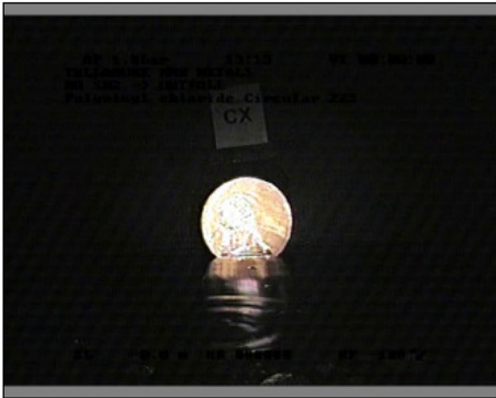
Photo: 3_1A 0m, Start node type, manhole, reference number : MH SW2
