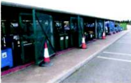
Images shows side access gates.
