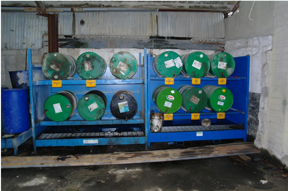
Photo 2 – Bunded Oil Drums in Maintenance Shed
