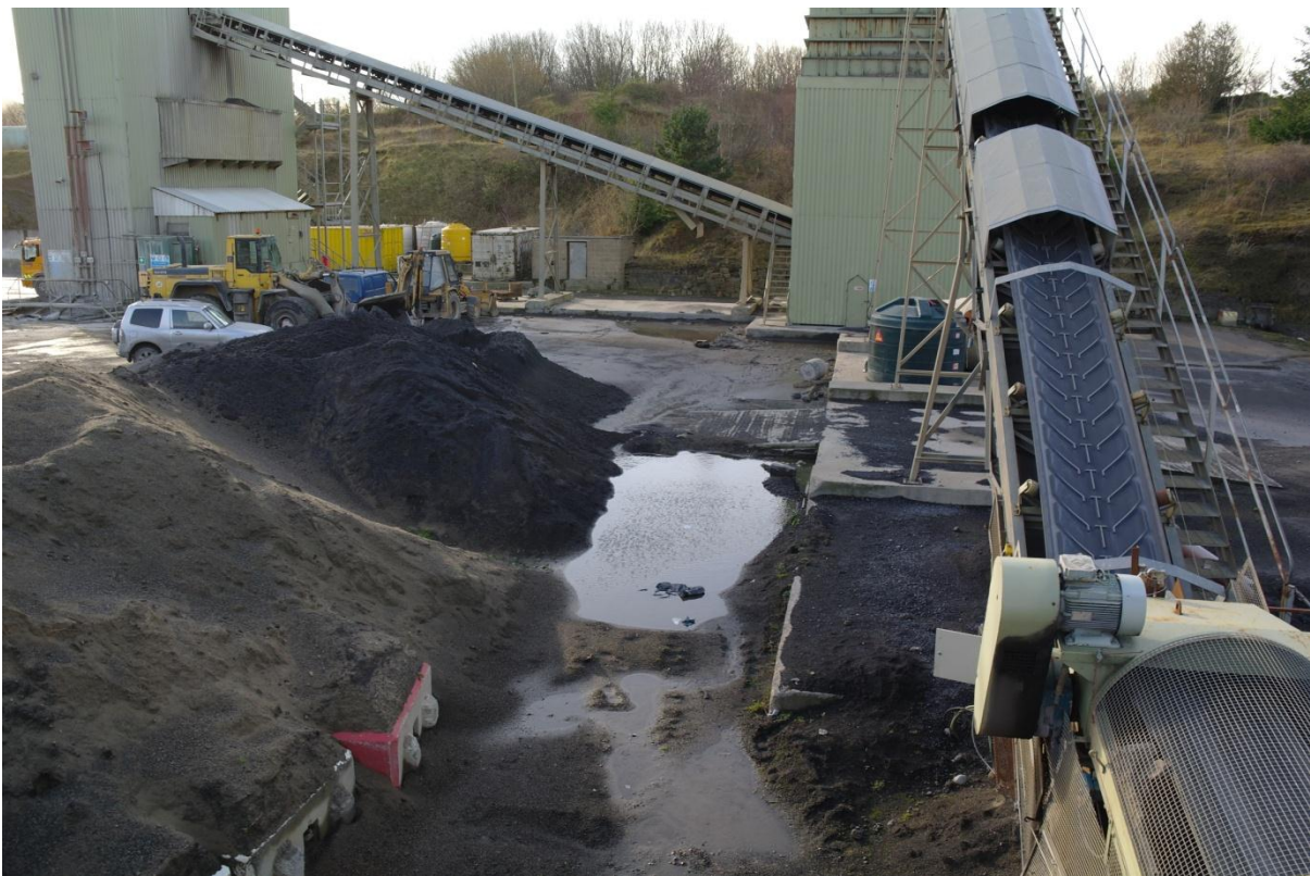
Photo 5 – Yard Drainage Impeded by Concrete Platform
