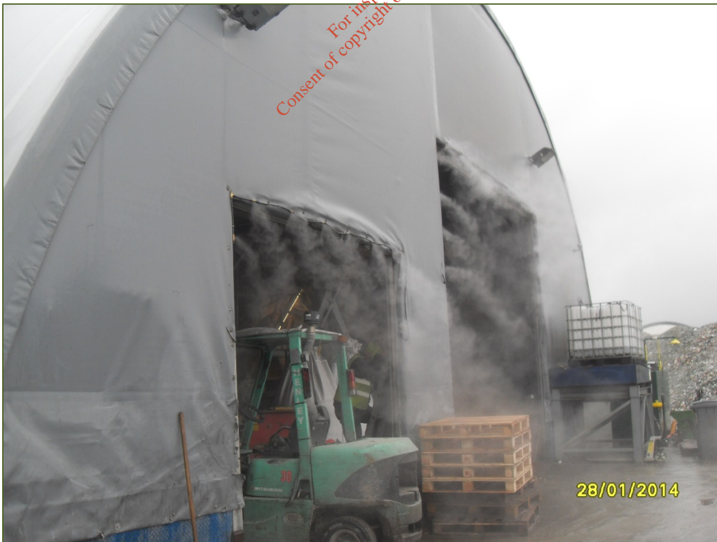
Photograph F.1.4: Misting system at Drying Plant (2)
