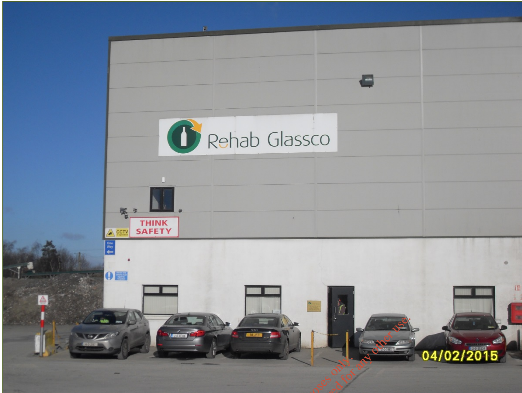
Photograph D.1.15: Site offices located at western side of Main Process Building
