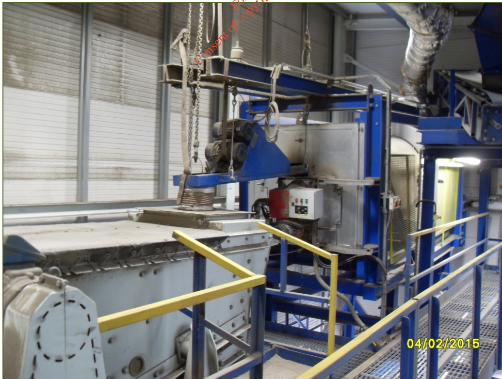
Photograph D.1.6: New fines processing line – interior (Main Process building extension)
