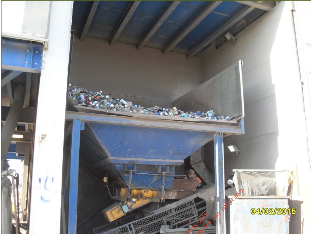
Photograph D.2.2: Glass loading into Main Process
