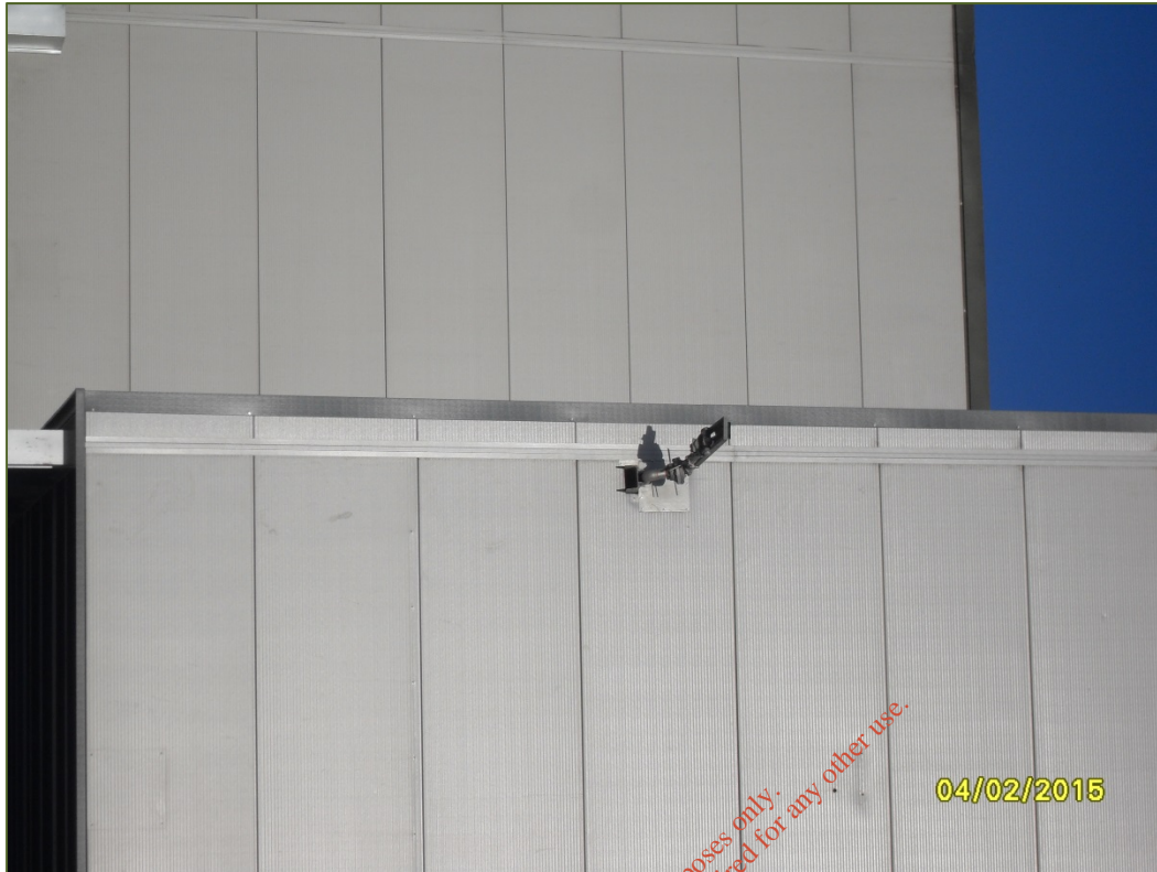
Photograph F.1.1: Water gun #1 positioned at Main Process building - extension
