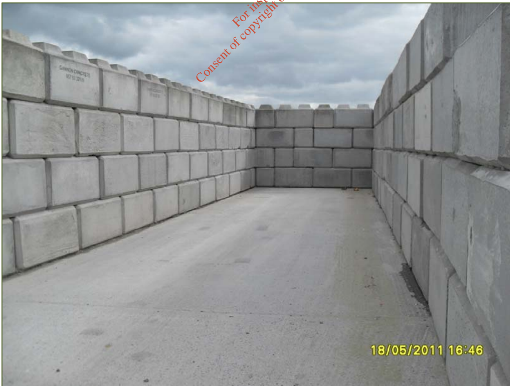
Photograph D.1.12: Storage bay
