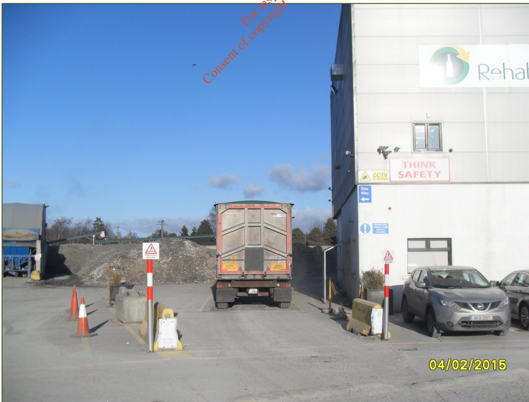
Photograph D.1.8: Weighbridge position and operator's window
