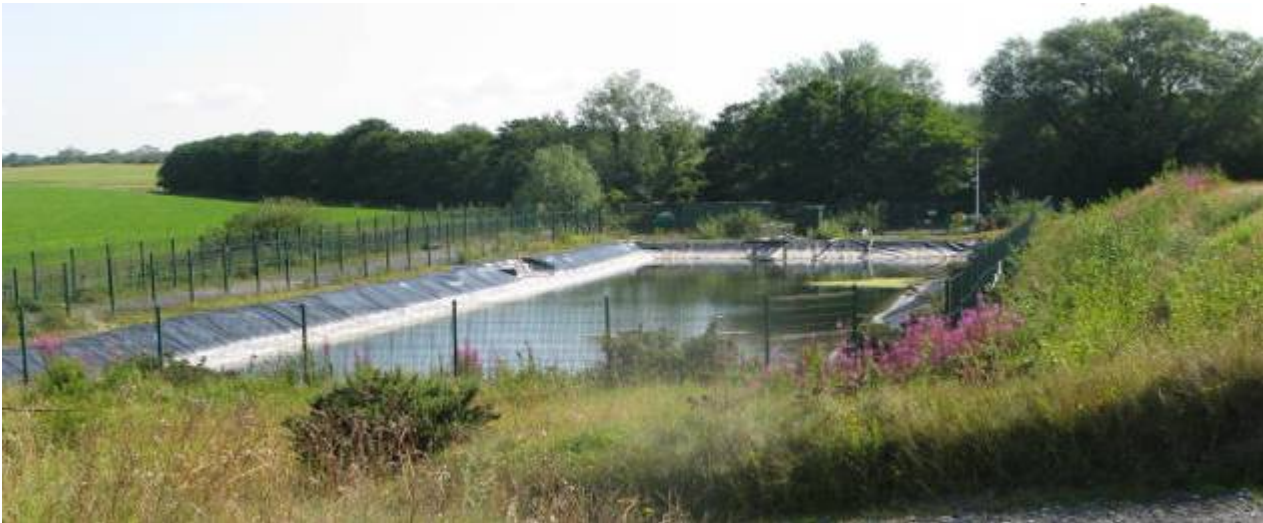
Figure 12.1: Existing Surface Water Attenuation Pond
