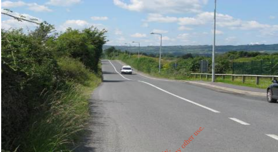
Figure 3.11: Local road outside Powerstown Landfill (looking west)
