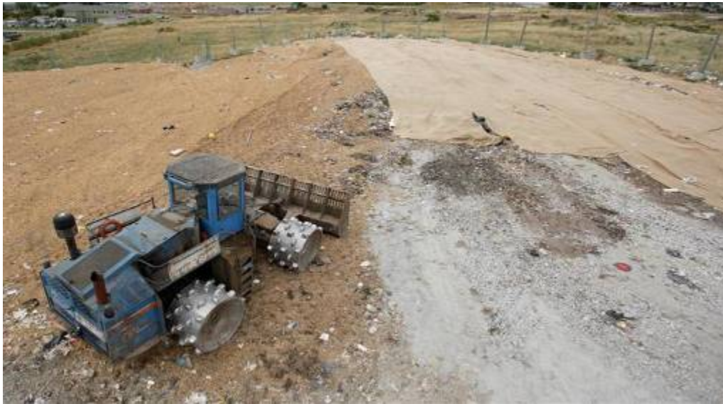
Figure 3.3: Typical landfilling operation using waste compactor
