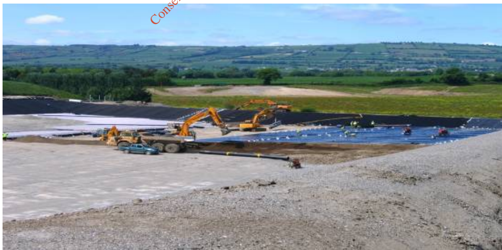
Figure 3.6: Cells 15-18 under construction in 2006
