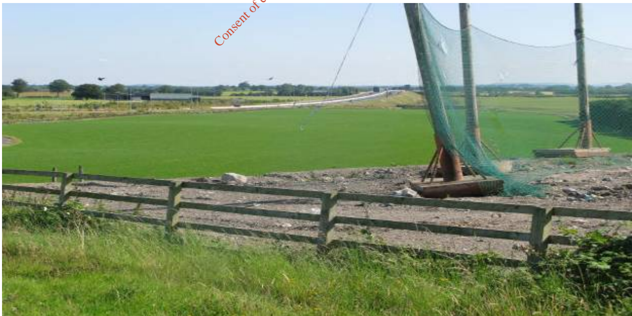
Figure 14.1: View from Phase 2 looking north west along the M9
