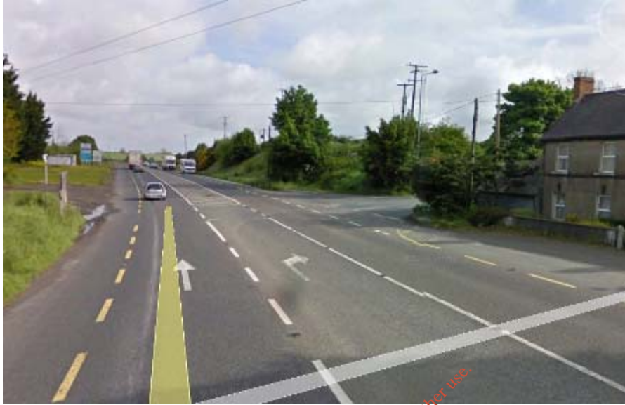
Figure 10.2: Photo showing Junction on R448 with L3045 leading to the Powerstown Facility (looking north)
