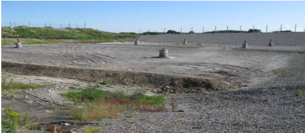
Figure 2.1: Cell 17 and 18 at Powerstown Landfill
