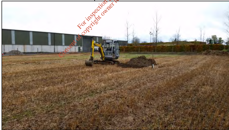
Trial pit as excavated on site.
