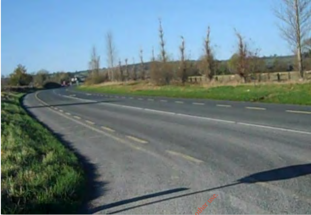
Figure 2.5 Visibility to left at Jock's Lane junction with N80
