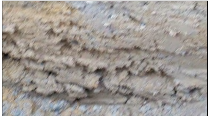
Soft Clay impermeable till material below 900mm.
