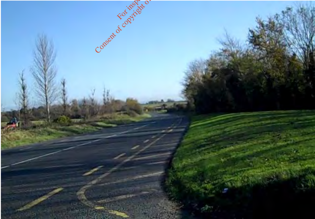
Figure 2.6 Visibility to right at Jock's Lane junction with N80
