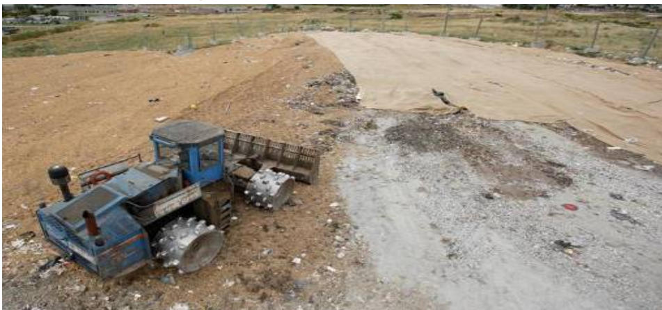
Figure 2.5: Typical landfilling operation using waste compactor
