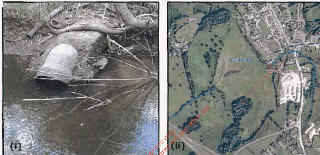
Figure 2.1: (i) Primary Discharge to Mill Stream and (ii) Typical Turlough characteristics in dry weather, picture taken in June 2010 (source: Clare County Council)
