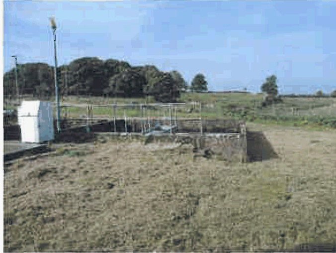
Photo 1: Existing Settlement Tank
