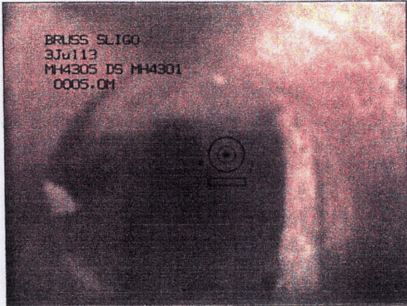
Photo: 7_5a, Tape No.: 1 5m, Joint displaced. Medium
