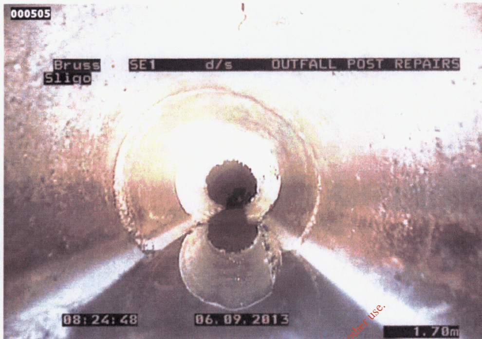
Fig 1,2 MH 4305 to MH 4294 2no dislocated joints - Liner inserts completed.
