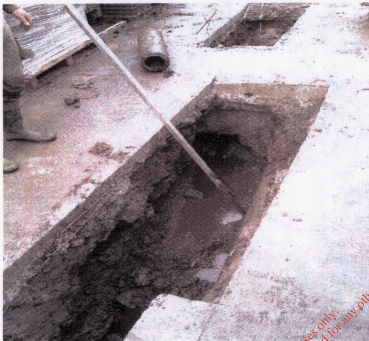
Fig 1,2 MH 4345 7m of pipework to be replaced
