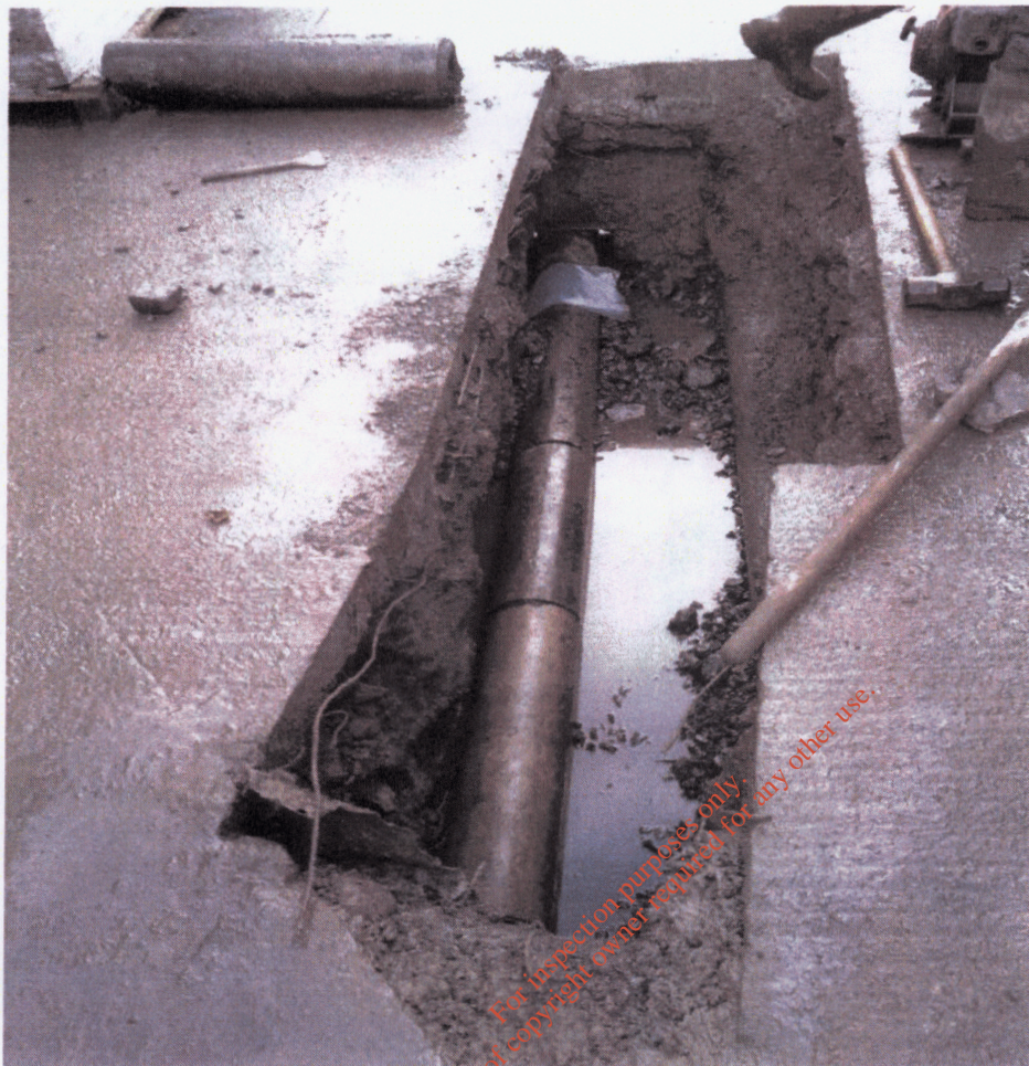
Fig 1 New Pipework in place – MH 4301 – MH 4345 7 m
