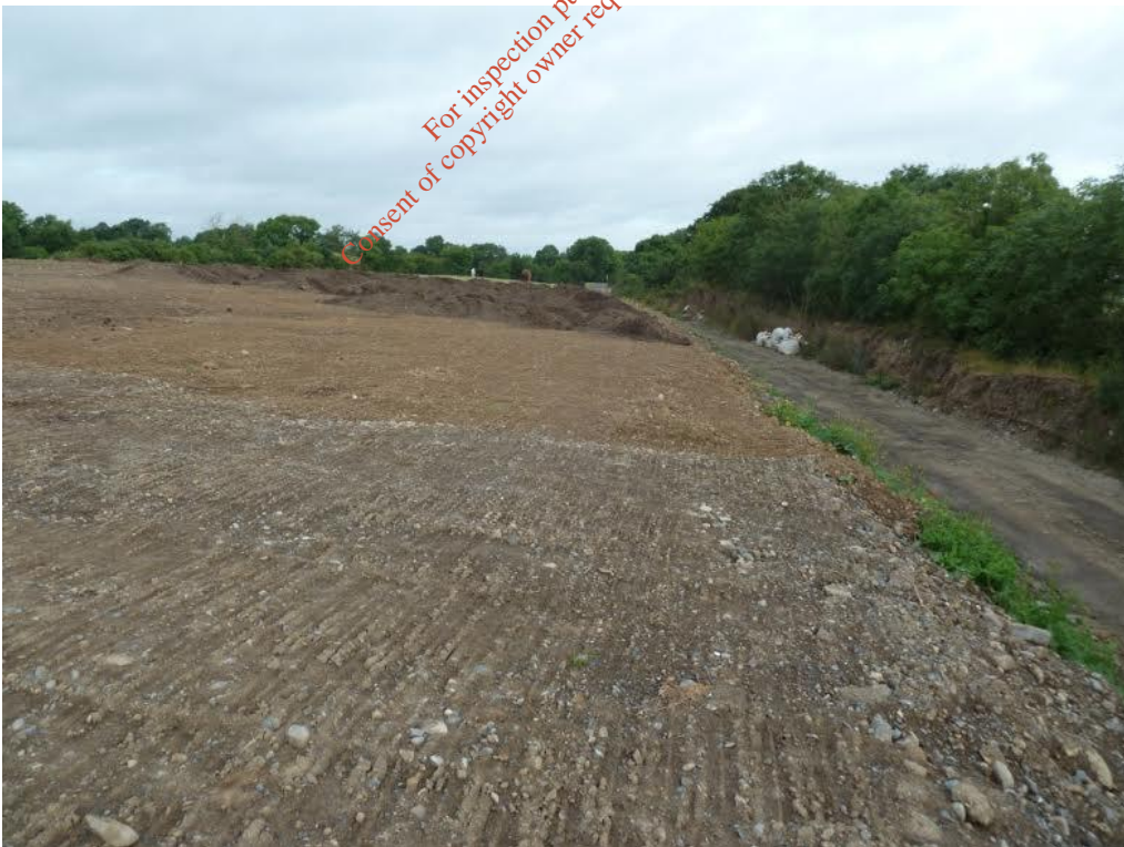
Plate 3.9.4: Northern end of proposed development area, looking north west
