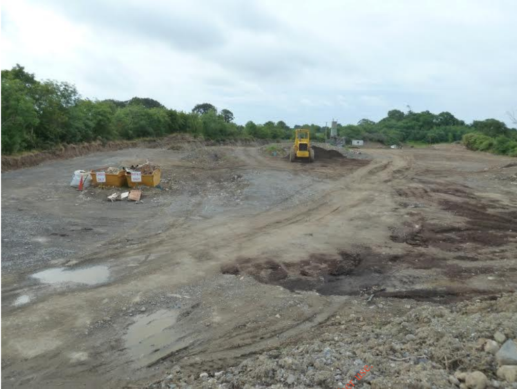
Plate 3.9.3: Middle of proposed development area, looking south
