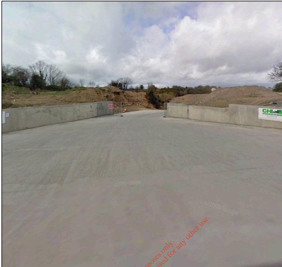
View 9: Looking North from L7526 Public Road into the new authorised Site Entrance for the Grannagh Recovery Facility.
