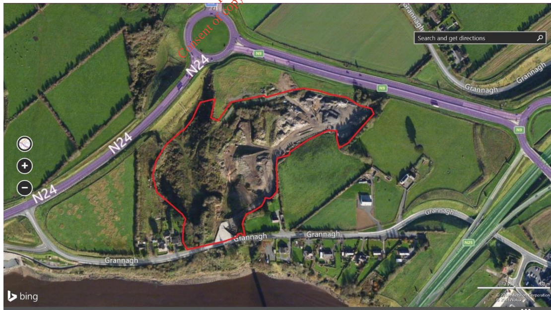
Recent Aerial Photograph of Site Showing Restored Eastern Section and New N24 Bisecting the Quarry Site (Source: Bing)
