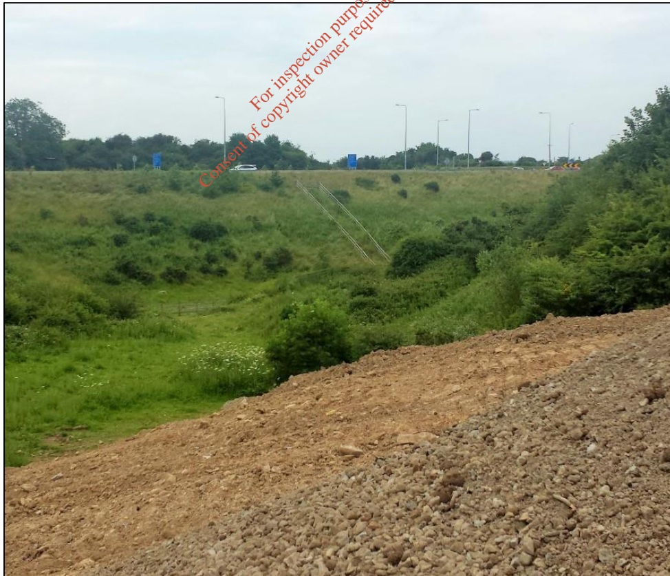
View 2: Restoration Works within Grannagh Site looking North to Granny Roundabout
