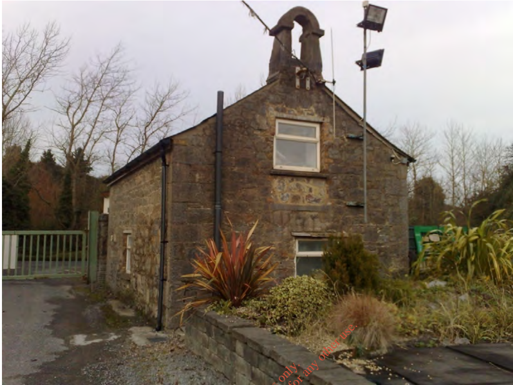
Plate 9.1 View of the Engine House at Milverton looking north.
