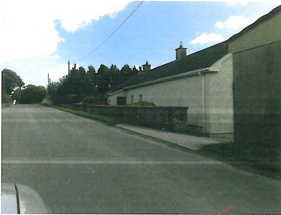
Fig. 11.4. View of structure 1 on Donore Road.
