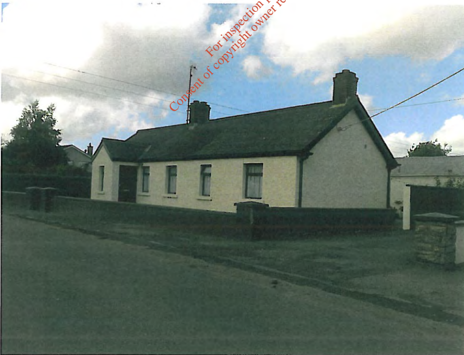
Fig. 11.5. View of structure 2 on Donore Road.
