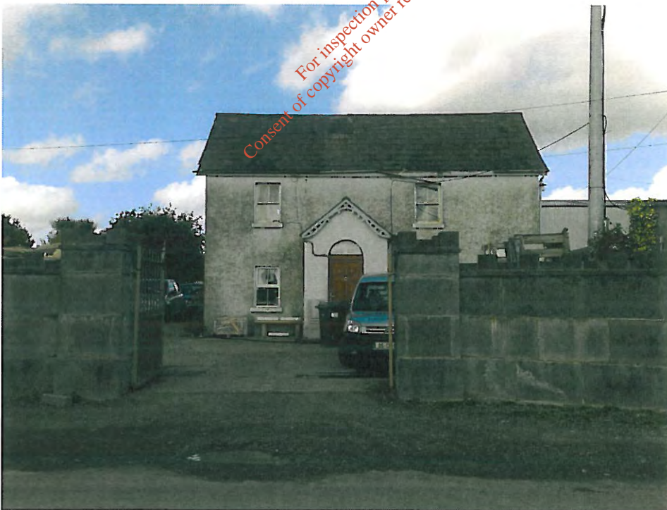
Fig. 11.7. View of structure 4 on Donore Road.
