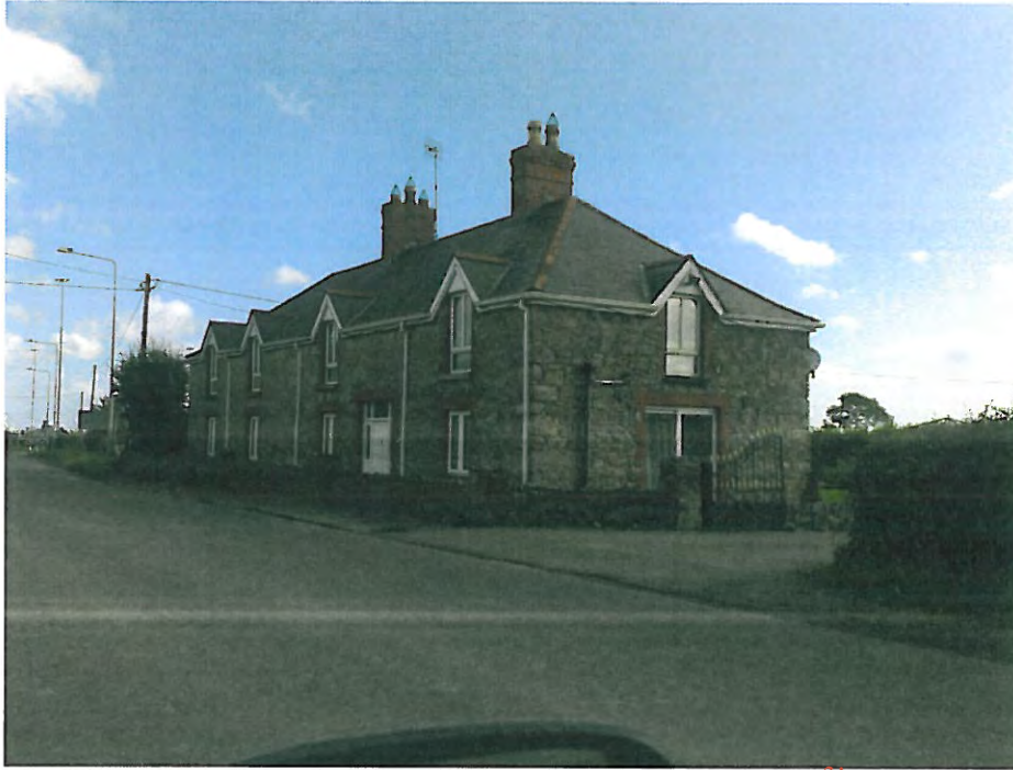
Fig. 11.6. View of structure 3 on Donore Road.
