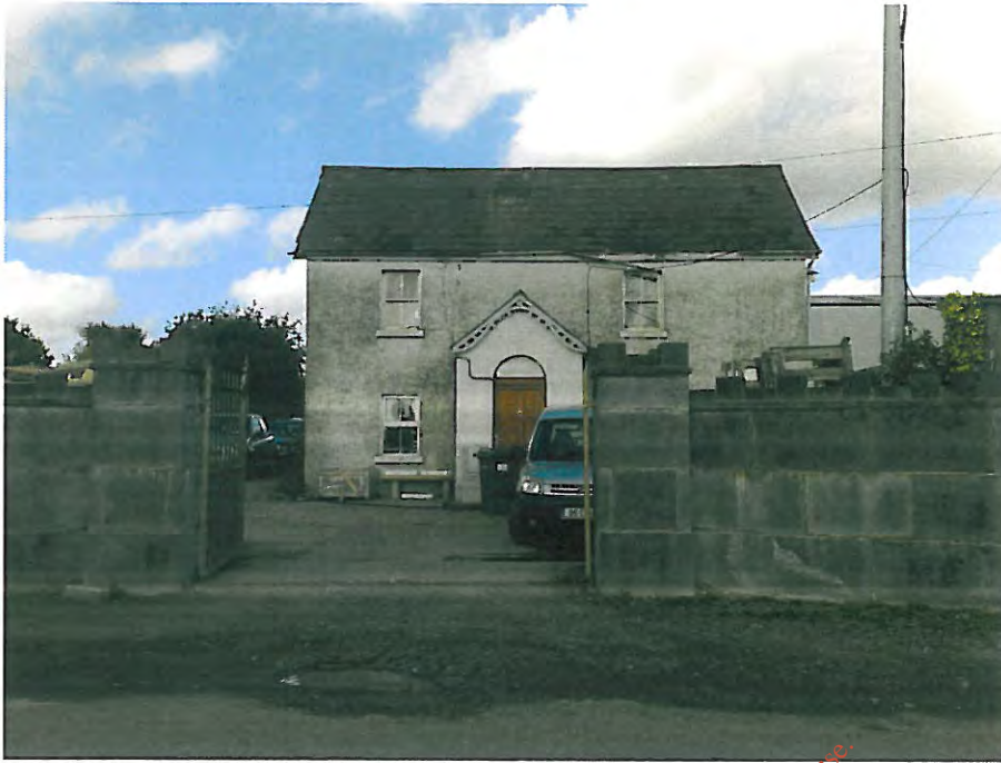
Fig. 11.8. Area 1 looking south-west across its length.
