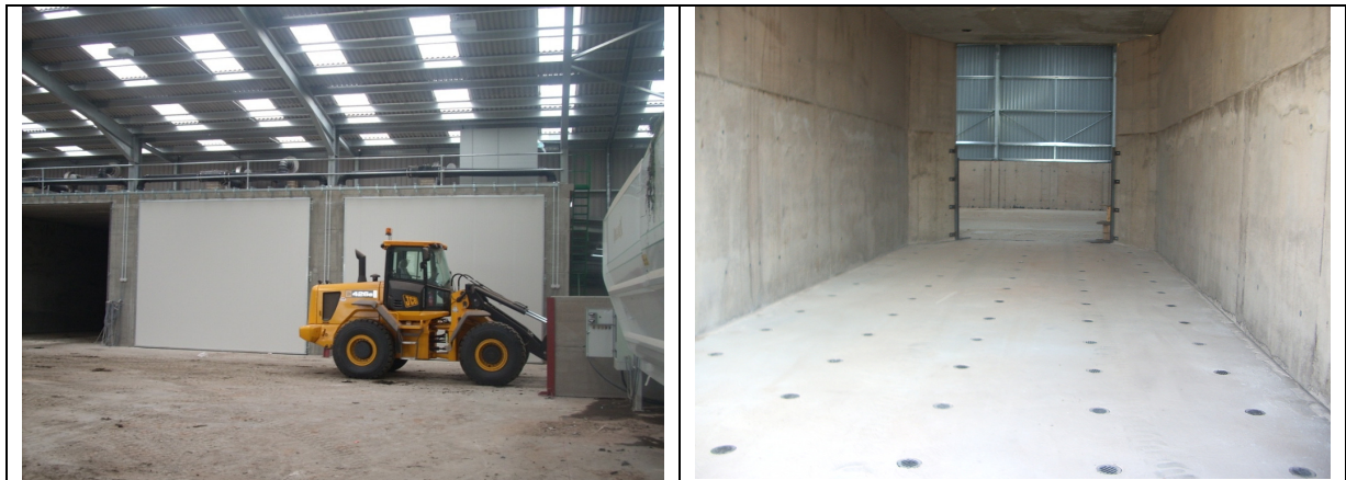
Figure 9 Exterior of the composting biocells illustrating the sliding doors (left) and the proprietary C:N in-pavement aeration system (right).
