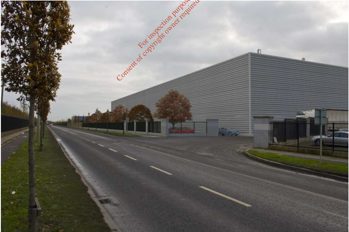
Photograph 3 : View of Proposed New Building (North West of Site Entrance)
