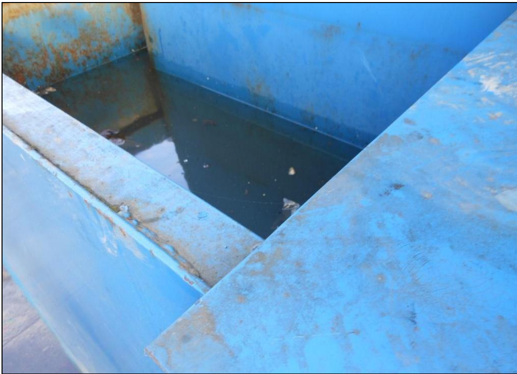
Photo 3 The bund during the hydrostatic test 20/11/12
