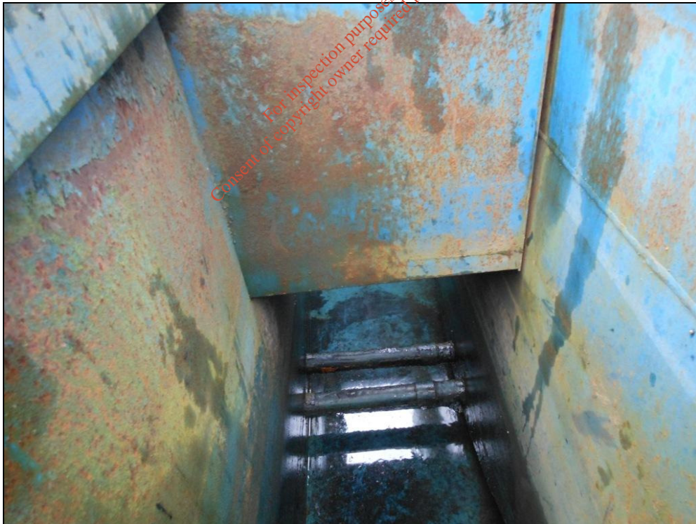
Photo 2 Inside the bund during the visual inspection on the 19/11/12
