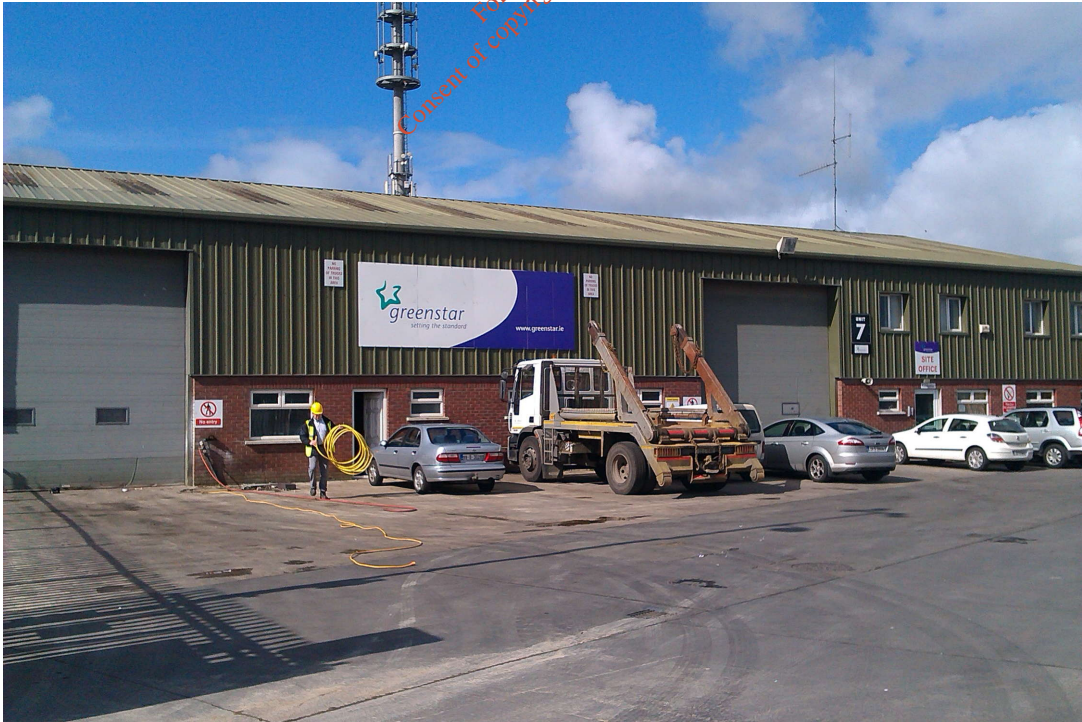
Photo 4 – Admin & Maintenance Building
