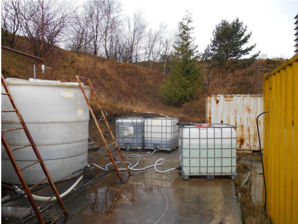
Figure 8 2 off unbunded IBCs by concrete plant
