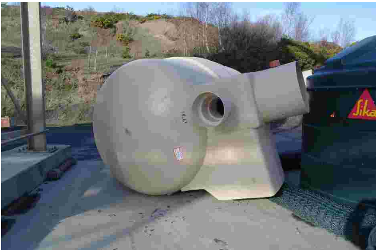
Photo 6 – Hydrocarbon Interceptor Awaiting Installation
