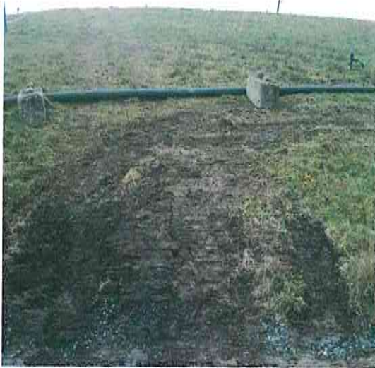
Plate 13 North East Slope
