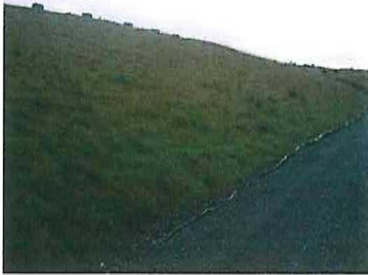
Plate 15 North West Slope facing south
