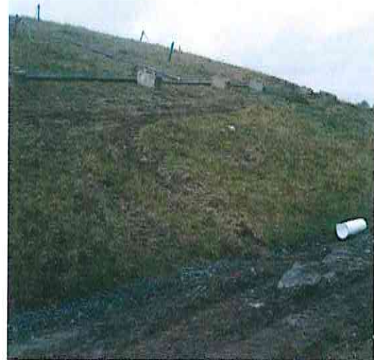
Plate 14 North East Slope
