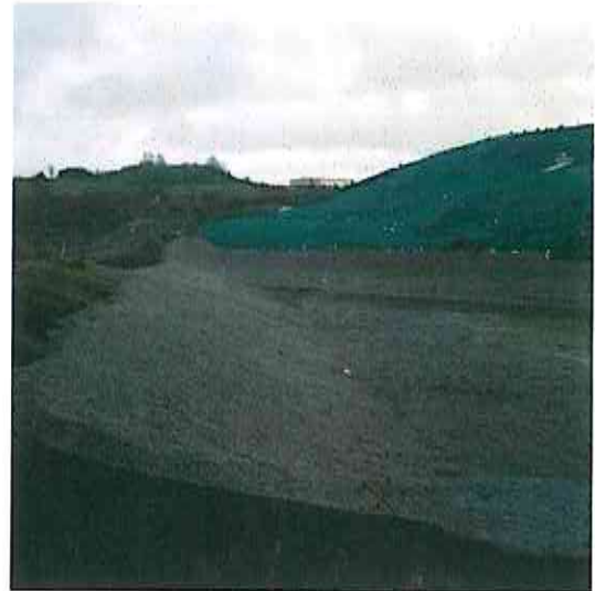
Plate 19 Cell 4 facing east
