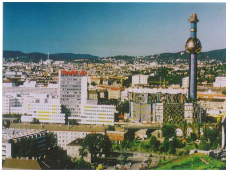
Incinerator in Vienna
