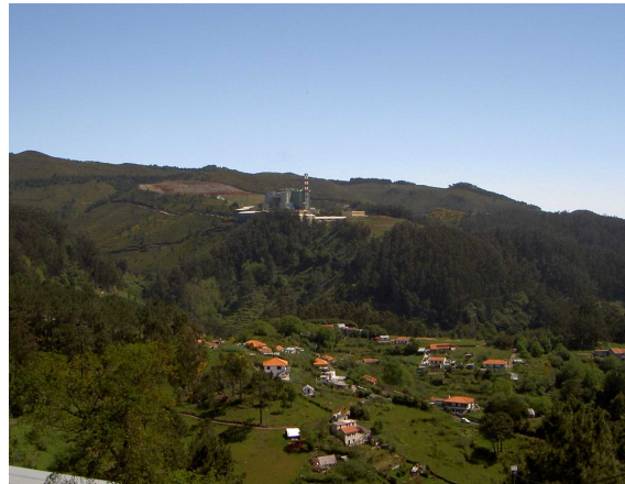
Waste-to-energy facility on Island of Madeira
