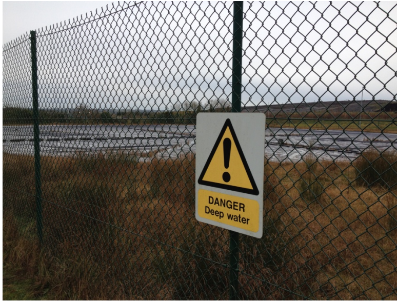
Figure 2.12: Perimeter Fencing with Warning Sign
