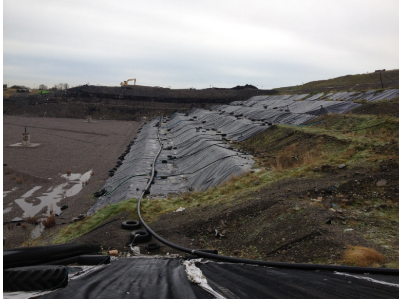
Photograph 24: Northern slope of Cell 9
