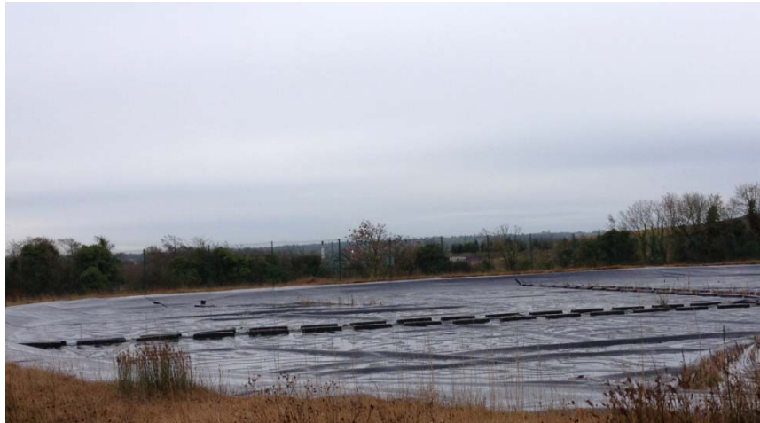
Figure 2.8: Leachate Lagoon Cover (looking West); Vegetation Growth
