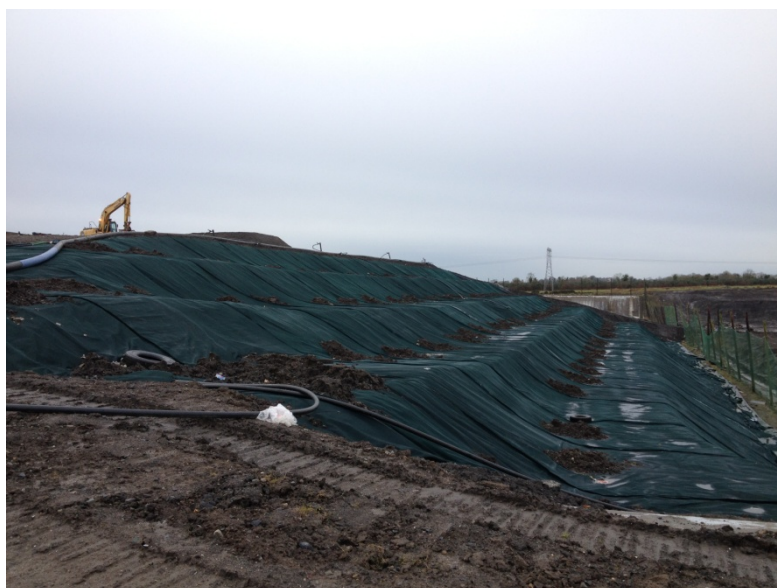
Photograph 25: Northern slope of Cell 12
