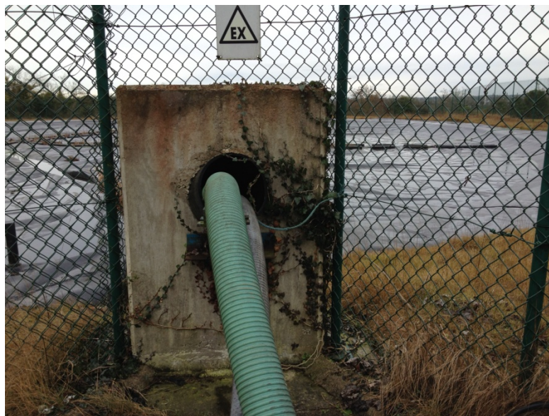
Figure 2.2: Extraction Pipe headwall; ivy growth
