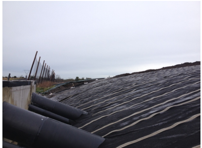
Photograph 23: Final Capped Area Awaiting Soils
