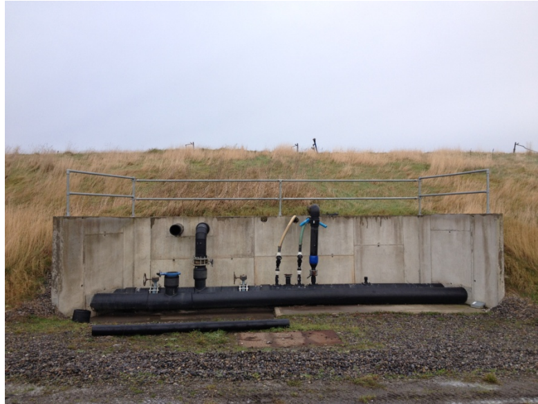
Photograph 26: Retaining Structures at Cell 1 & 2
