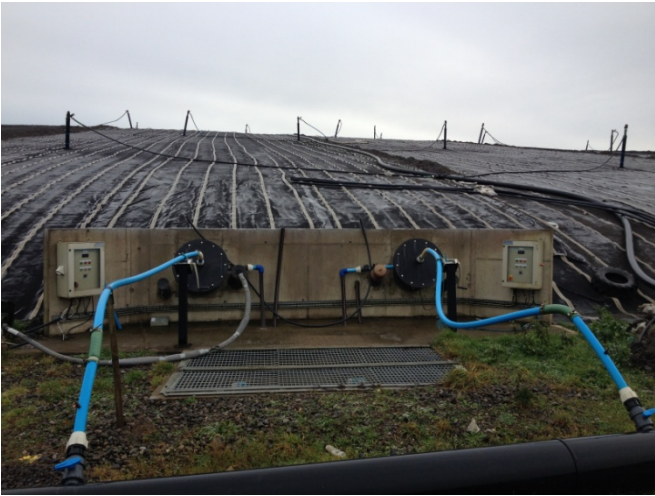
Photograph 8: Headwall at Cells 5 & 7
