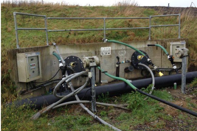
Photograph 4: Headwall at cells 2 & 4
