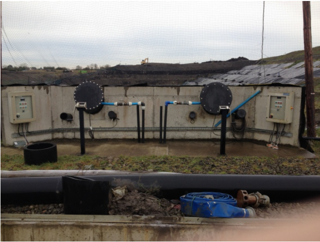
Photograph 15: Headwall at Cells 9 & 11
