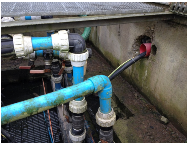
Photograph 6: Concrete damage (construction stage finish)
