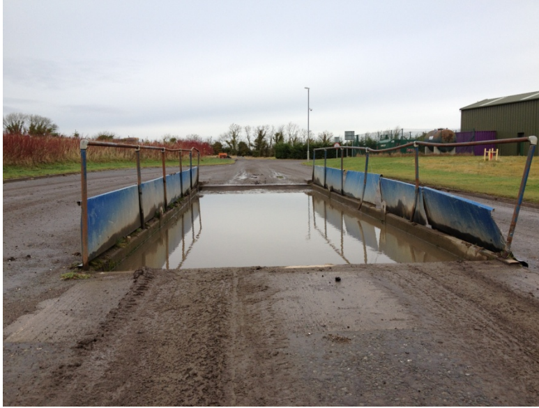
Photograph 19: View of wheelwash, looking North
