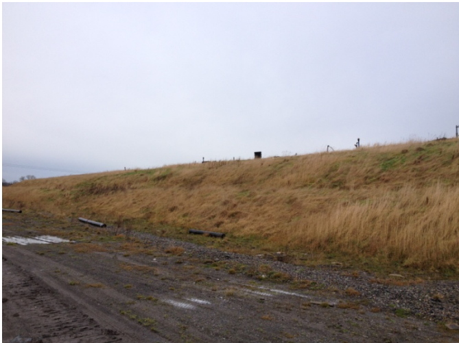
Photograph 22: Final Capped Area
