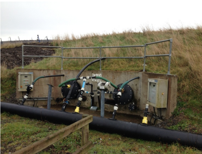
Photograph 1: Headwall at cells 1 & 3
