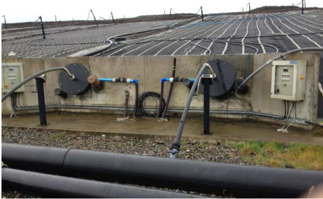
Photograph 11: Headwall at Cells 6 & 8
