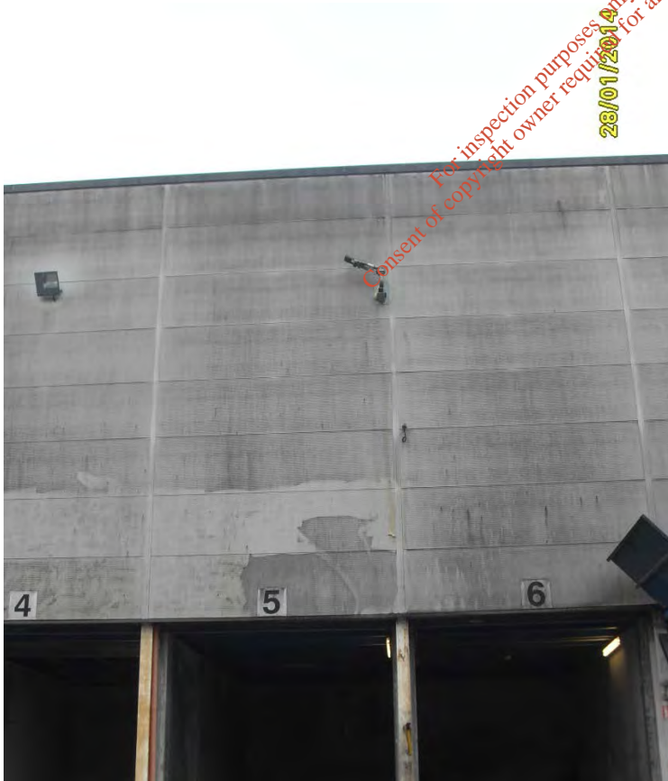
Photograph 2: Water gun #2 positioned at Main Process building
