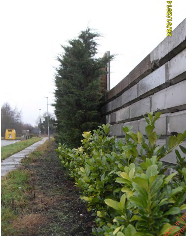
Photograph 12: Noise barrier and boundary planting adjacent to neighbouring property (2)
