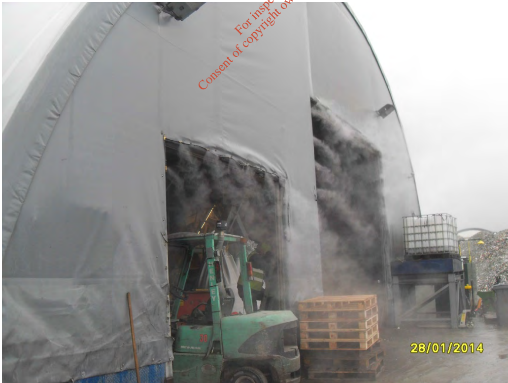
Photograph 4: Misting system at Drying Plant (2)
