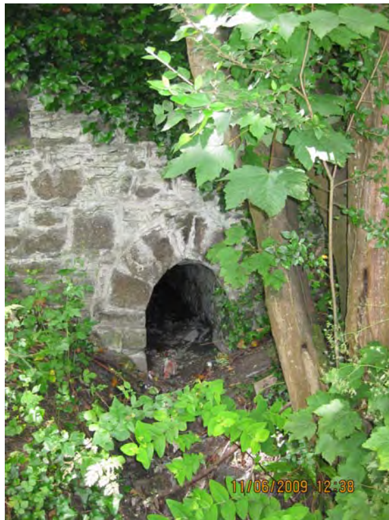
Fig. 22 SWO 15: surface water culvert combined with foul sewer overflow
