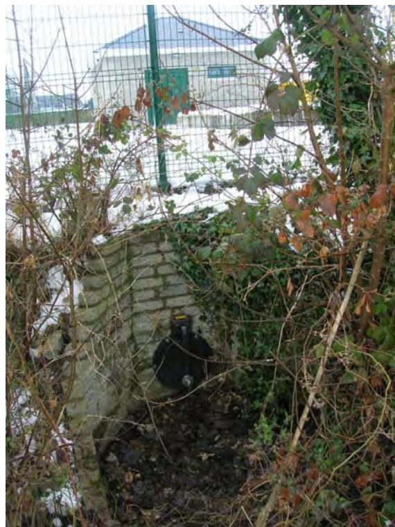
Fig. 21 SWO 14 – outfall and pumping station site
