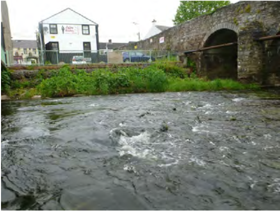
Plate 1. Site U2 at Celbridge Bridge.
