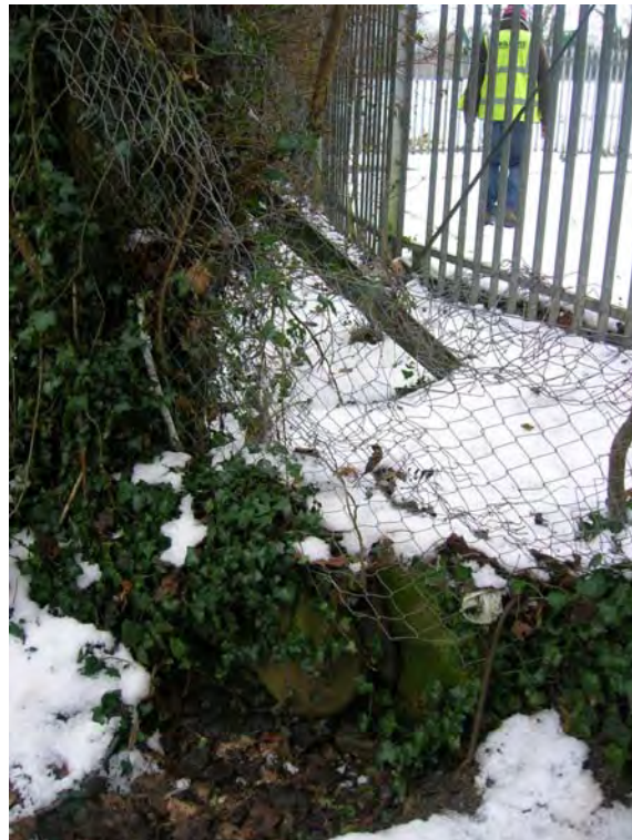
Fig. 17 SWO 6 – outfall at pumping station site
