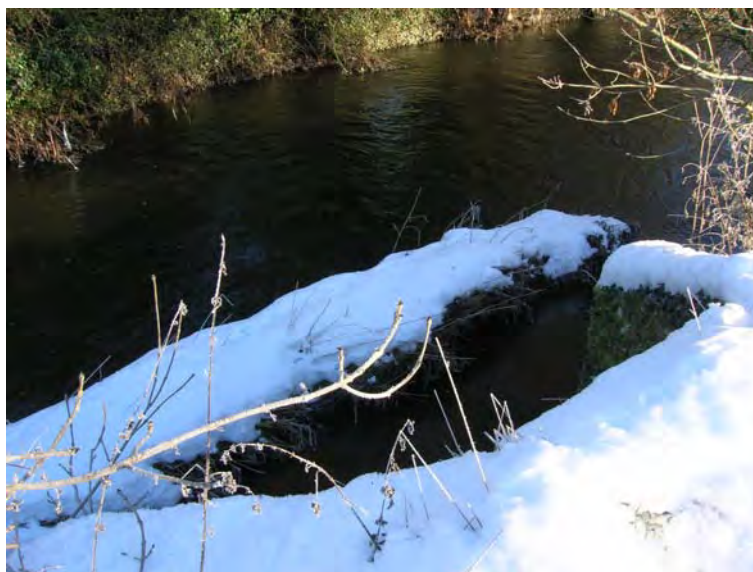
Fig. 8 SWO 4 – headwall structure at outfall to the river
