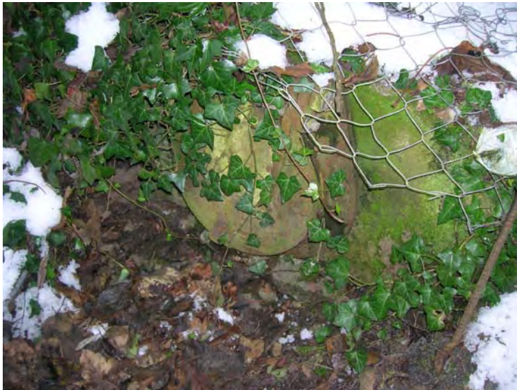
Fig. 16 SWO 12 – flap valve at outfall pipe
