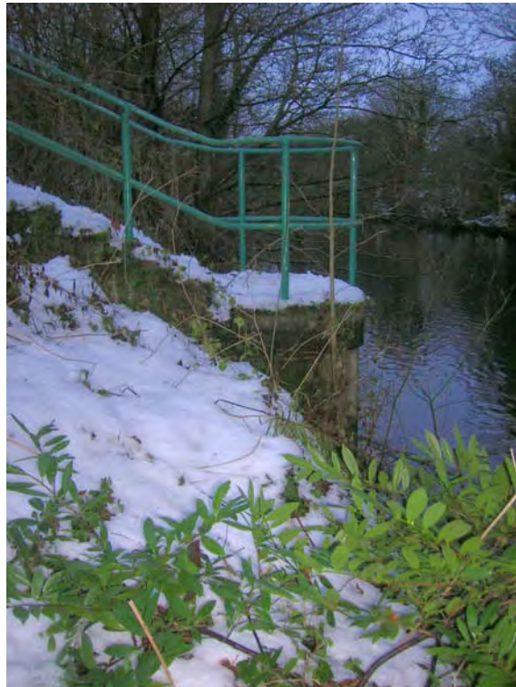
Fig. 1 SWO 2: outfall chamber visible from river bank
