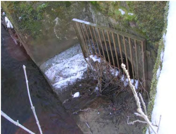
Fig. 7 SWO 4 – grating at outfall to the river
