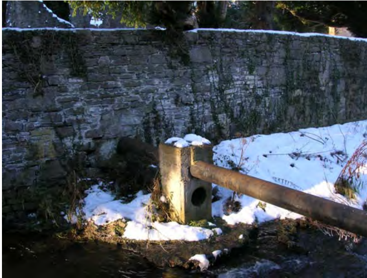
Fig. 9. SWO 5 – outfall to Lyreen Stream (open pipe at the bottom)
