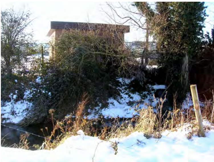
Fig. 4 SWO 4 and old pumping station, visible from opposite river bank
