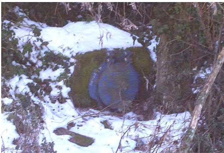
Fig. 3 SWO 3 – outfall with flap valve, located on Rye Water river bank
