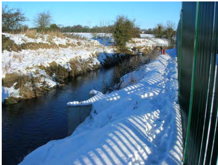
Fig. 6 Storm water overflow to Rye Water at new Kilcock Pumping Station
