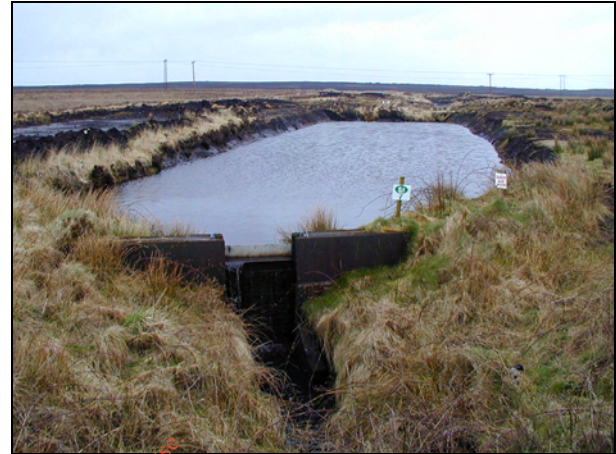
Plate 3.2 Bord na Móna Oweninny Works showing silt pond viewed from N59 North West of the ESB Power Station. The weir is at downstream end of lagoon.
