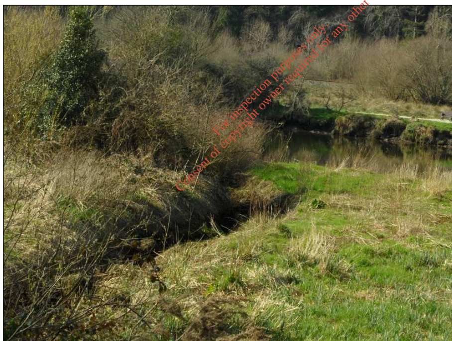
Plate 20 One of many drainage channels which intersect the floodplain between the N11 and the river corridor. These were characteristically overgrown and silted.
