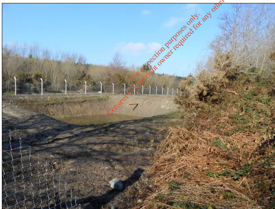
Plate 6 Recently constructed settlement ponds at the south western corner of the Brownswood Quarry site. The surface water from the quarry void will be discharged via a series of these settlement ponds to the cSAC.
