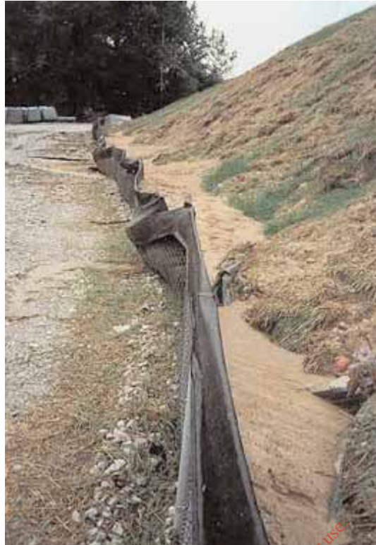
Image 5.2: Example of silt fence at toe of stockpile (source CIRIA Report No. C648, 2006)
