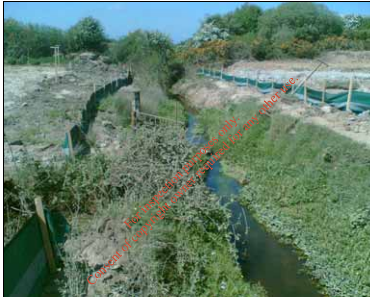
Image 5.1: Example of silt fencing on banks of watercourse (source CIRIA Report No. C648, 2006)
