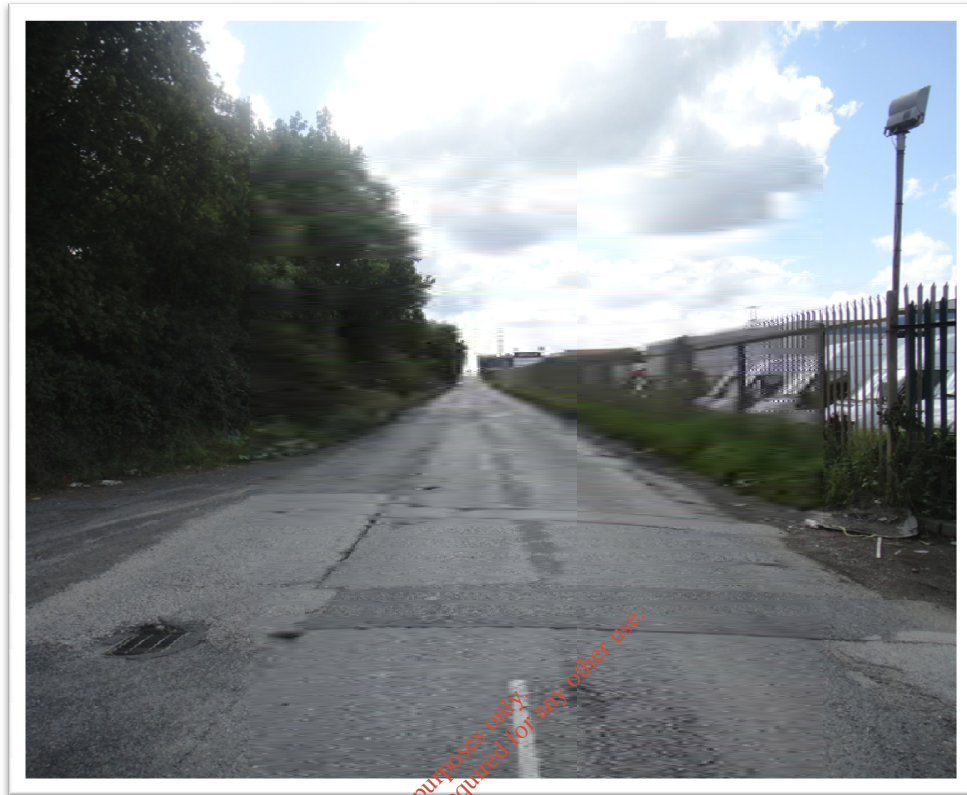
Plate 13-4 Kilshane Road near western quarry entrance
