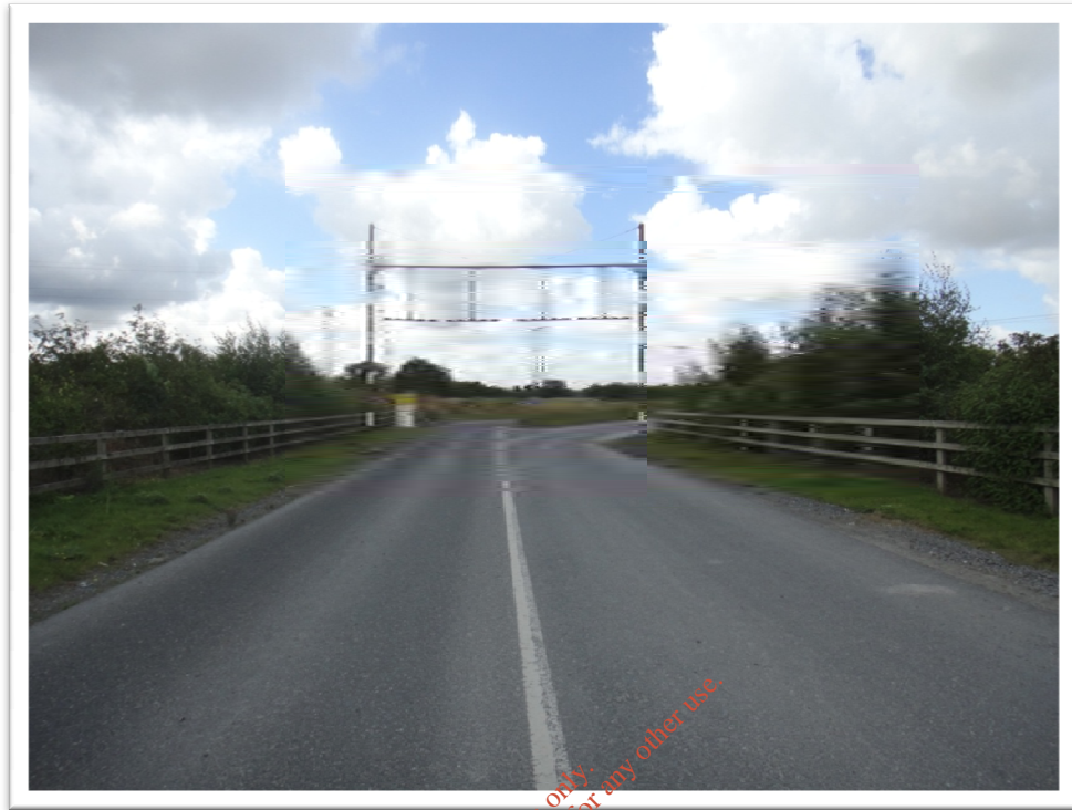
Plate 13-1 Access road from North Road to Huntstown Quarry
