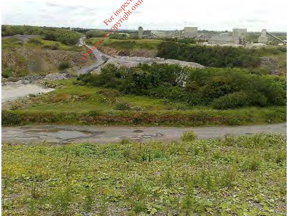
Plate 11.4 View of Central Quarry area 3 looking north.
