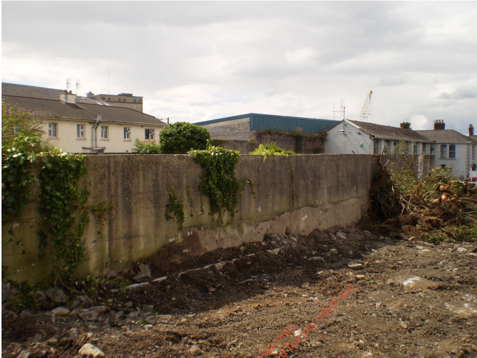
Photo 39) Tank 1 bund exterior
