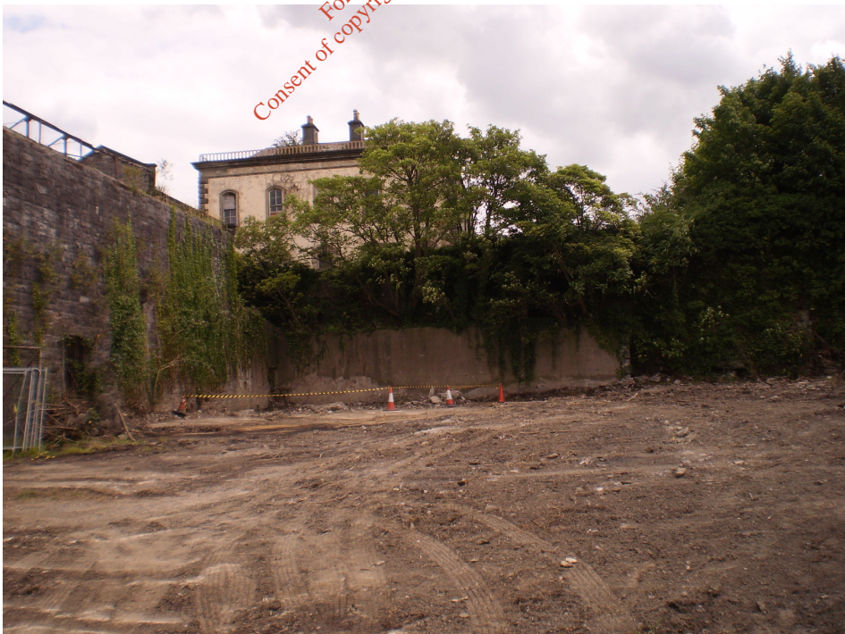
Photo 32) South west side of No.5 stores
