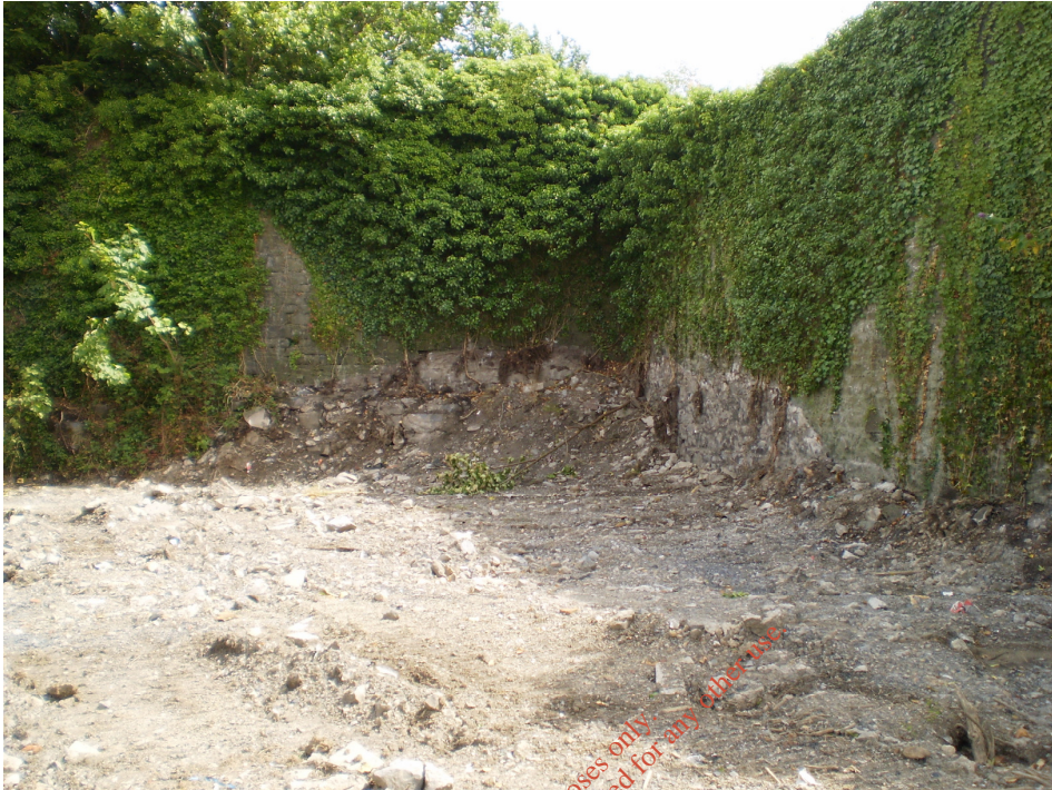
Photo 37) Site corner from Gasholder 3
