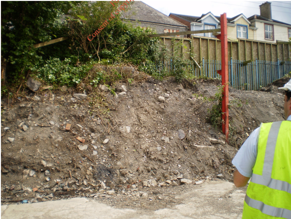
Photo 28) North eastern boundary
