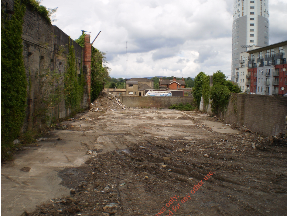
Photo 21) View towards Gasholder 1
