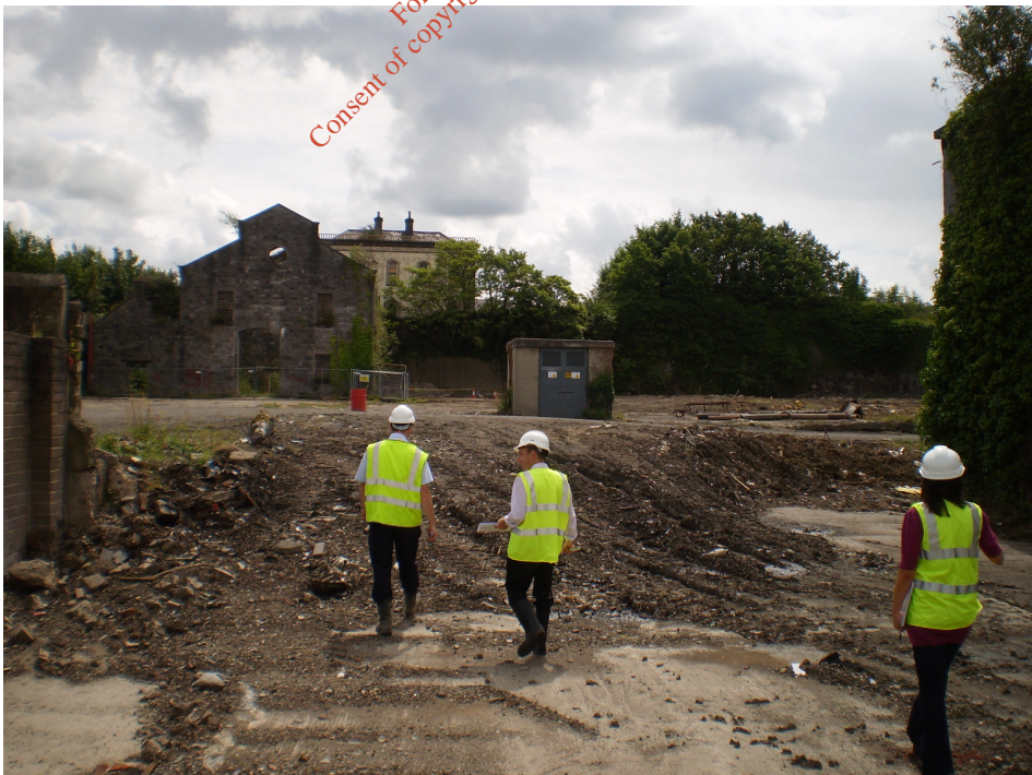
Photo 24) View towards ESB substation
