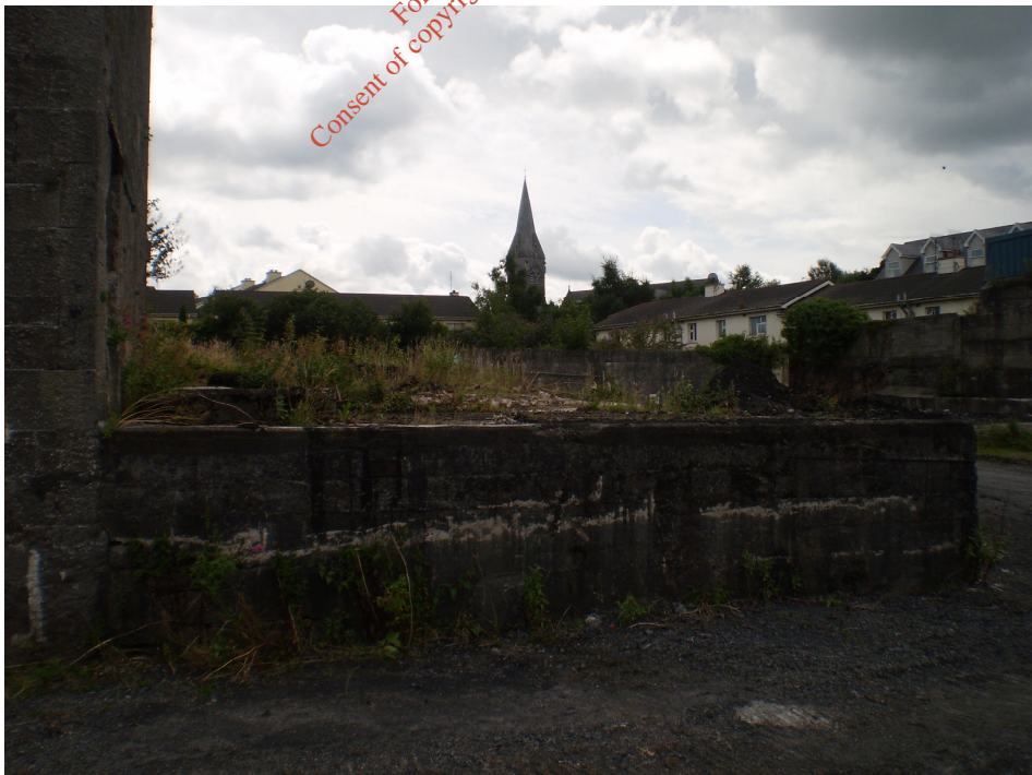
Photo 10) Booster house slab
