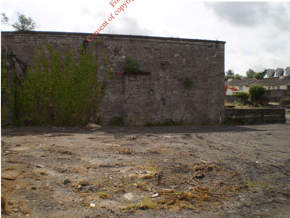
Photo 4) Back wall of booster house
