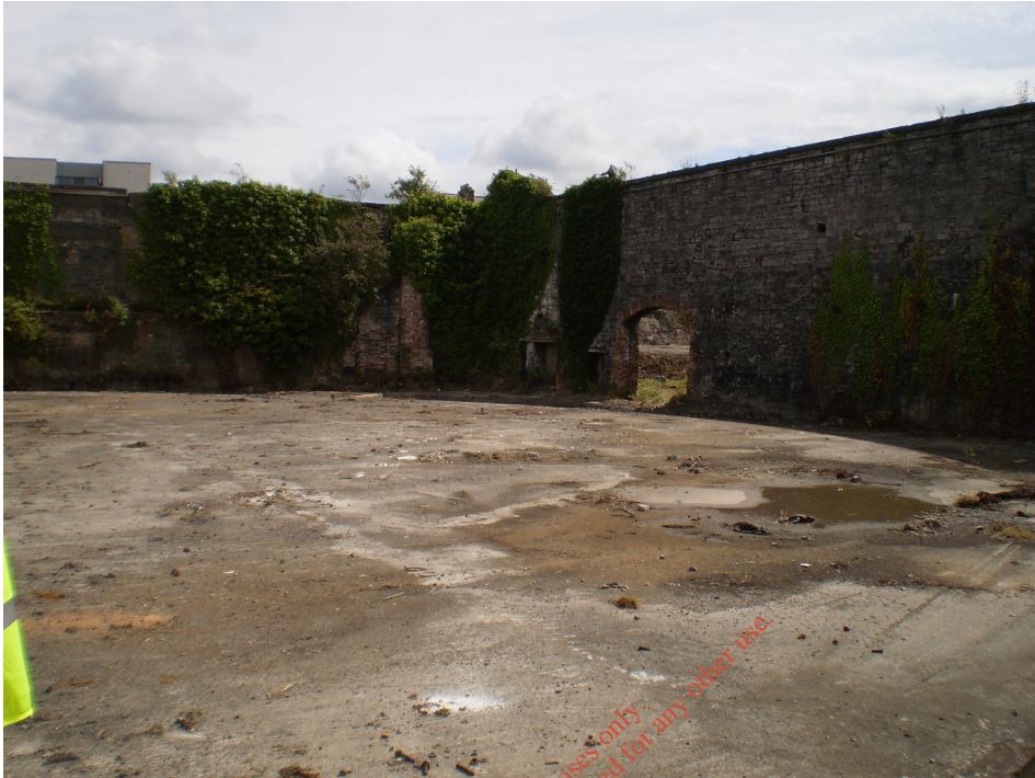
Photo 5) Looking west from Gasholder 2
