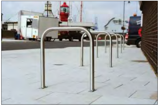
Proposed Cycle Stands - Sheffield Type Cycle Stand Cycle Stands Not To Scale
