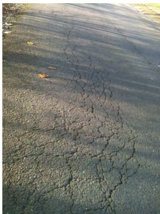
Plate 8.1: Alligator Cracking
