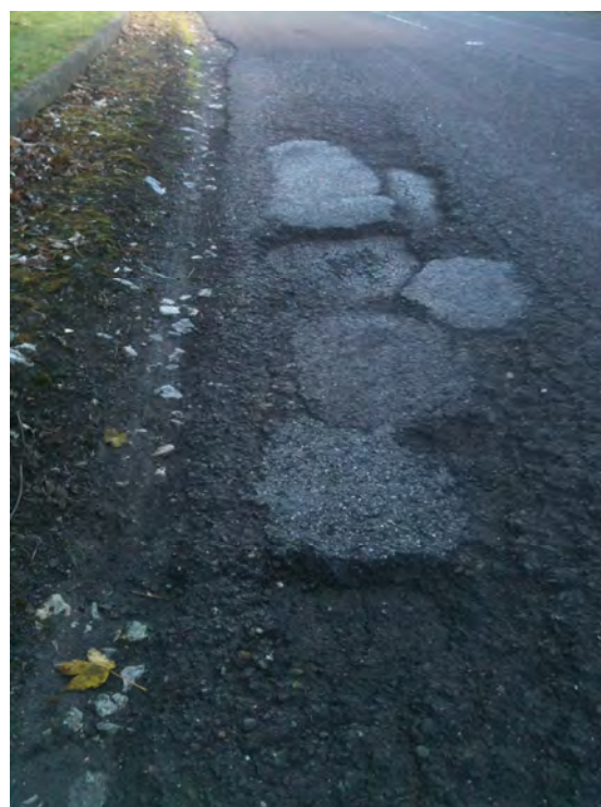
Plate 8.2: Potholing and Patching
