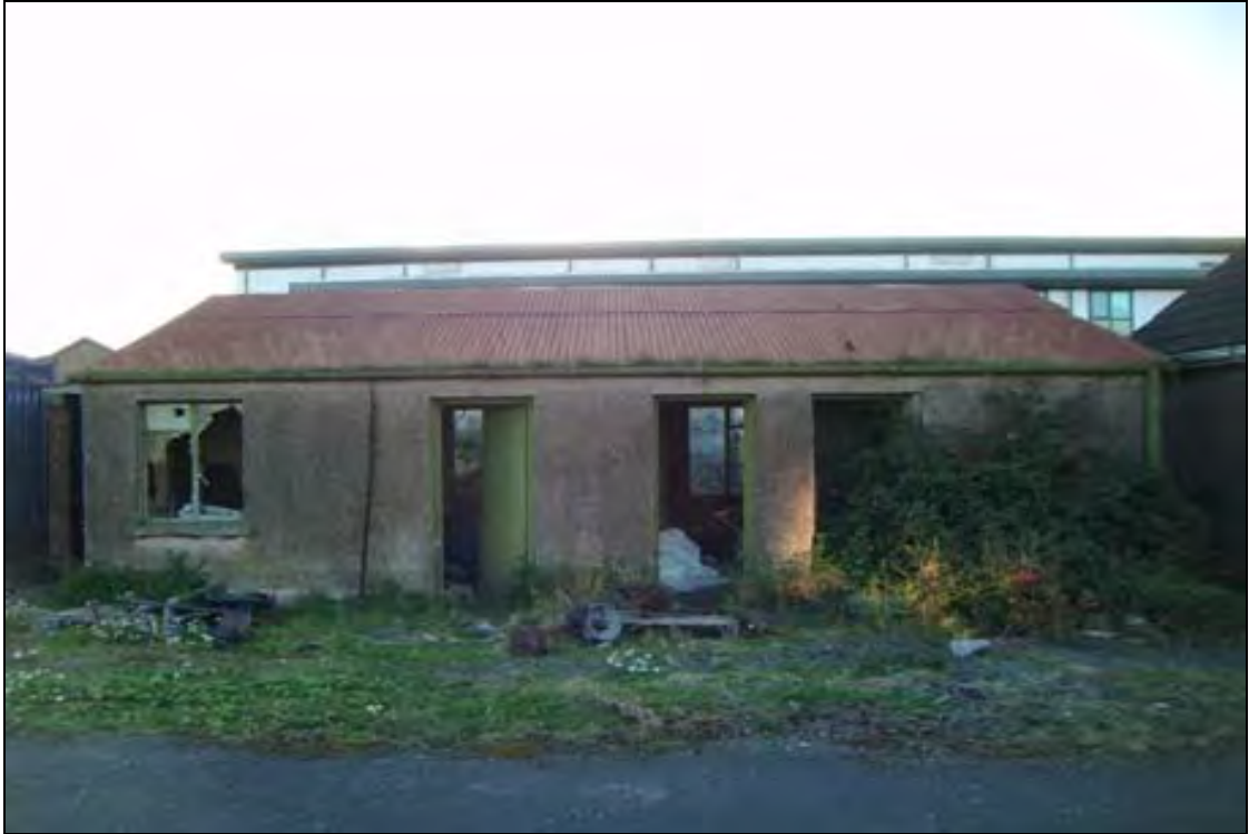
Plate 5: Derelict single-storey building
