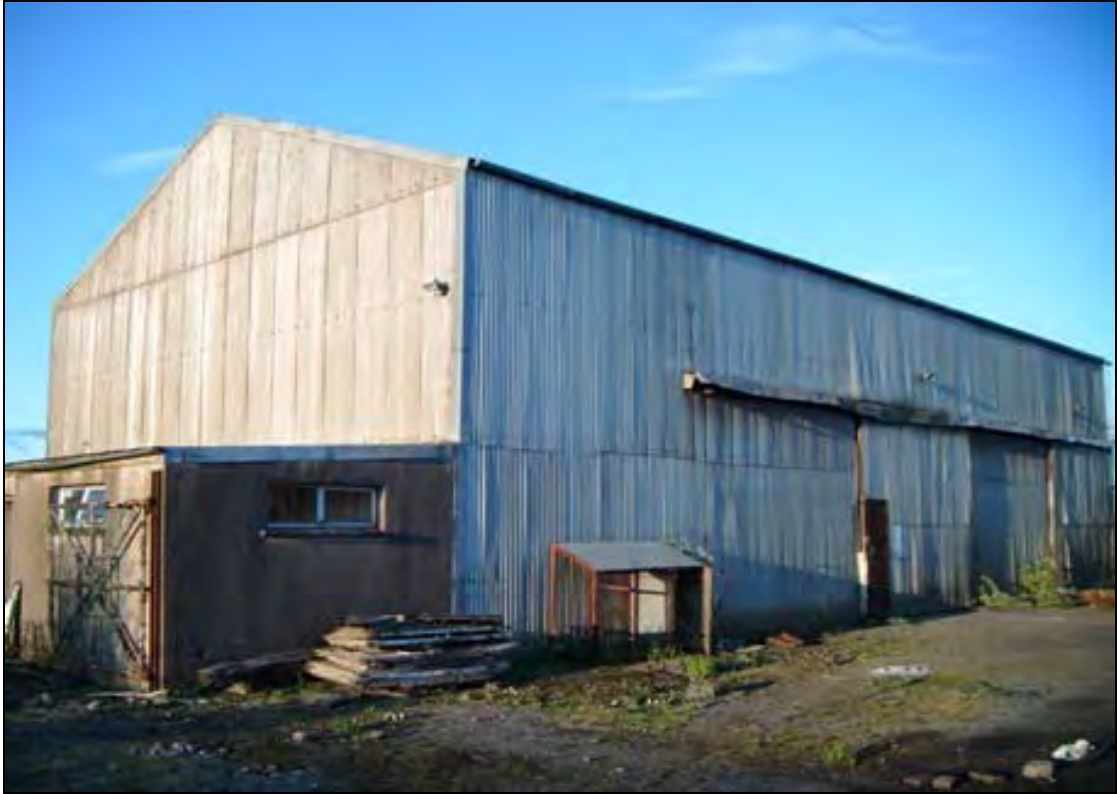
Plate 7: Large steel and iron maintenance shed which is still used for storage
