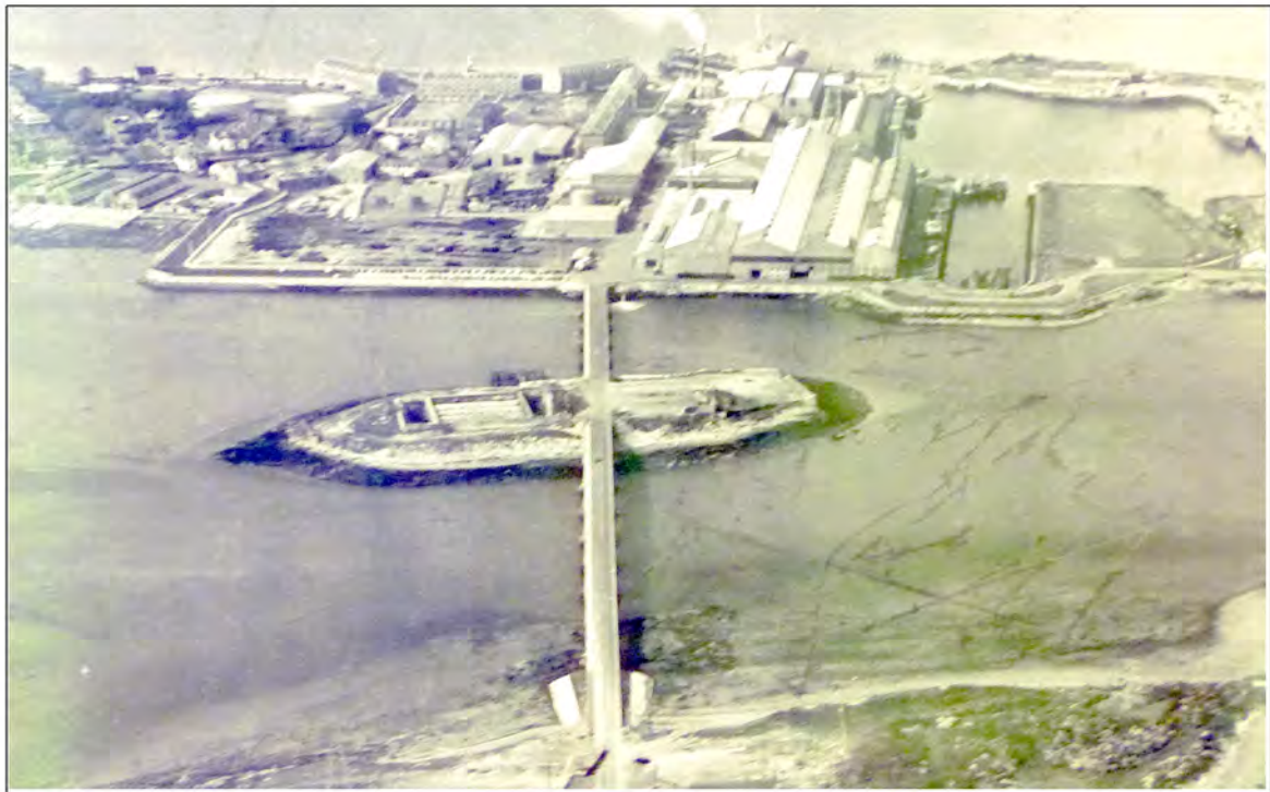
Fig. 15.10 Aerial photograph taken sometime in the late 1960's/ early 1970's before the demolition of the Steel Processing Plant
