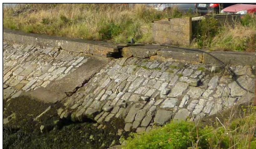
Plate 15.6 Rudimentary steps in the southeastern sea wall known as the 'Priest's Stairs'
