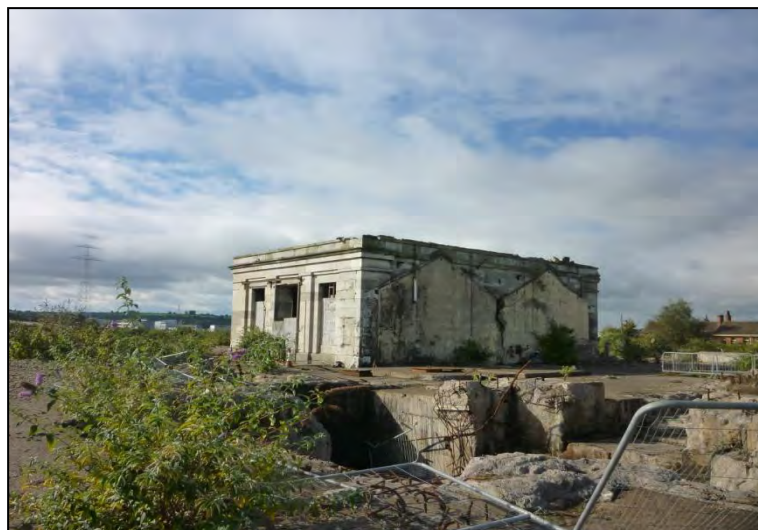
Plate 15.12 Pump house associated with the Naval Dock
