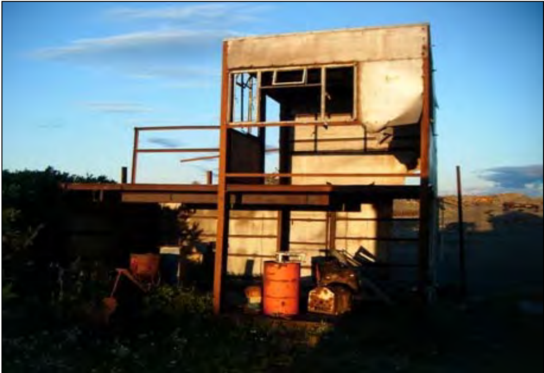
Plate 9: Small, derelict office constructed of steel and iron
