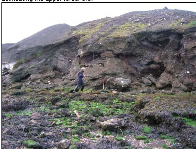
Plate 19: West-facing view of upper foreshore and large mound of slag material forming upper foreshore (1m scale).
