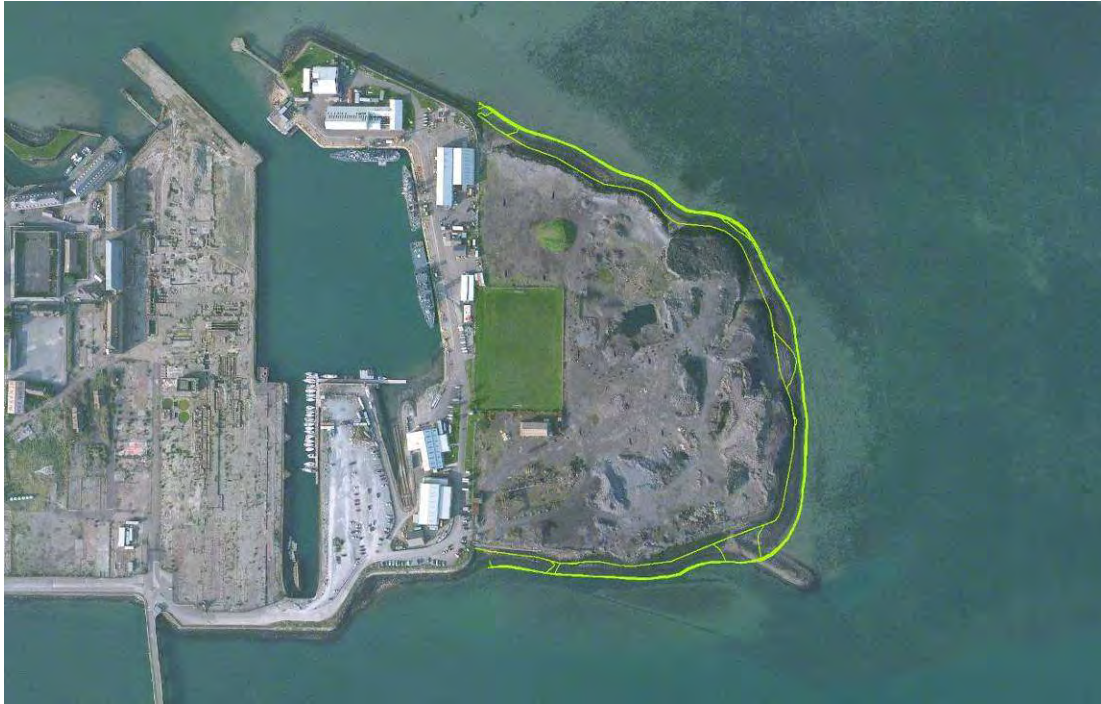
Figure 2.3: Extent of the bulk excavation of waste from Scenario B
