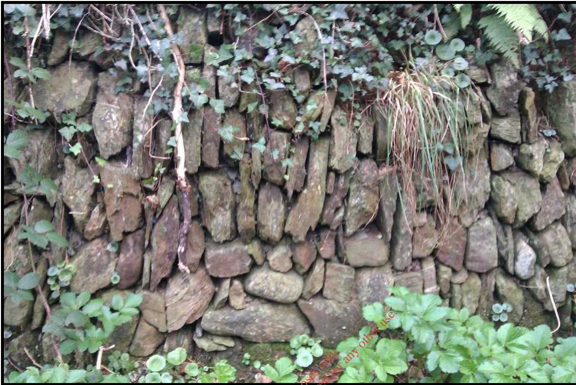
Plate 8 Drystone walling revetment of embankment along laneway
