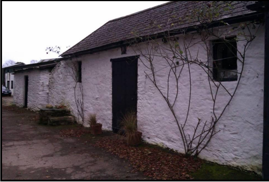
Plate 6 Looking west at outbuildings
