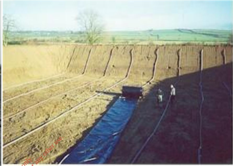
Installation of Geo-textile
