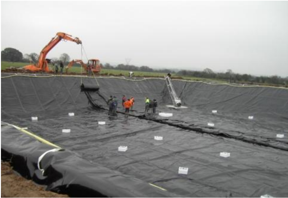
Installation of Integrity Pipe-work under Geo-textile
