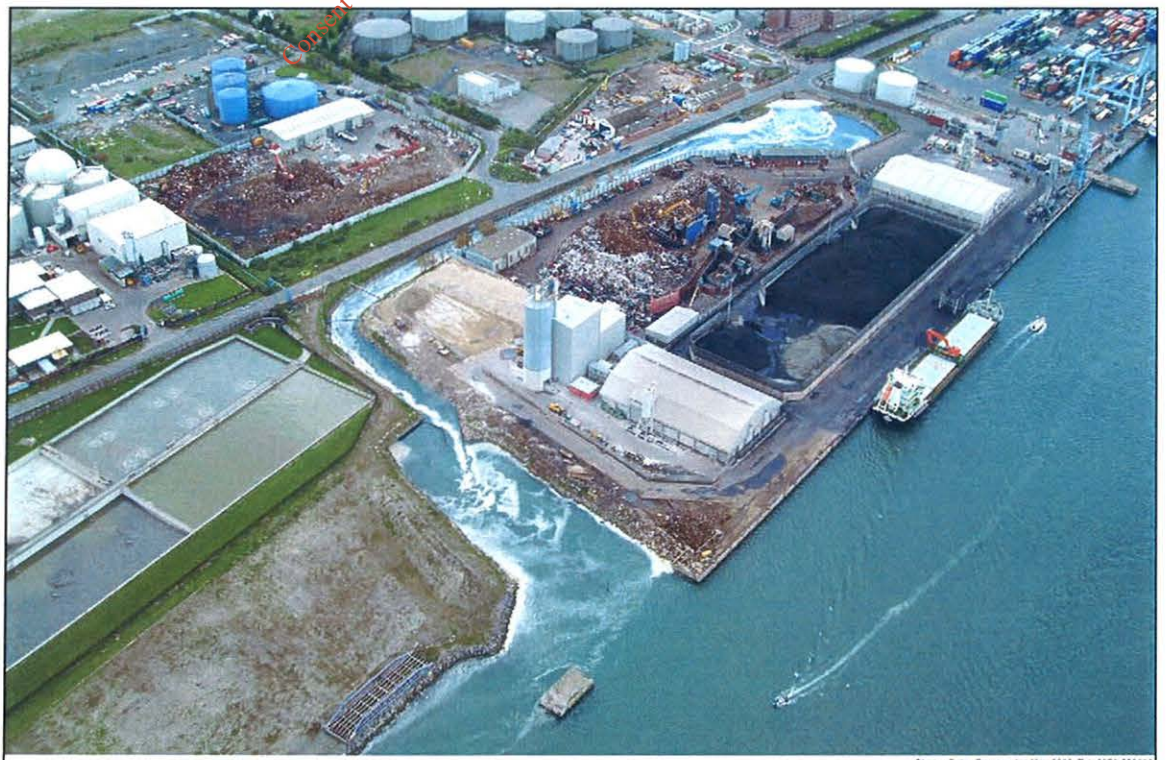
Plate 6 Aerial View of the proposed WtE facility site from the northeast
