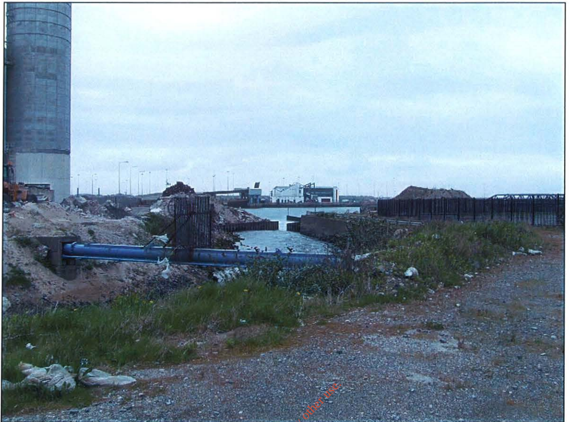
Plate 5 Watercourse to the north of the proposed WtE facility site
