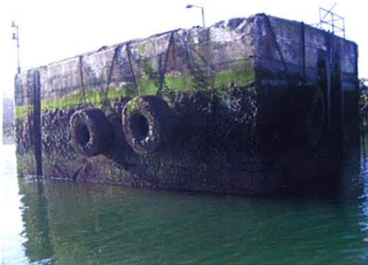
Plate 5.15 The structure of site Lb.
