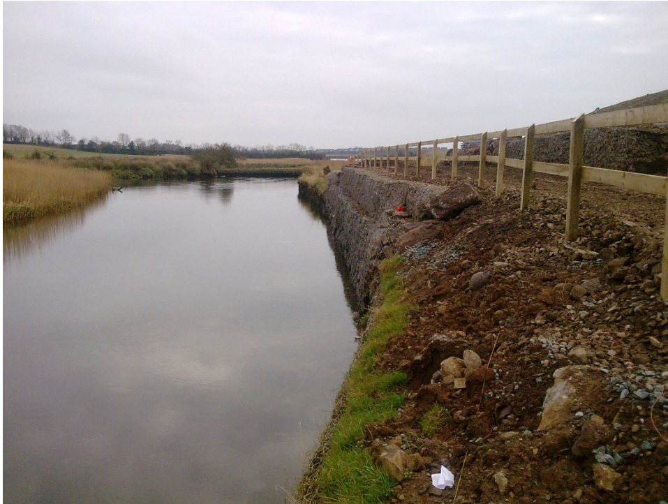
The River Colligan and bank protection works at the landfill
