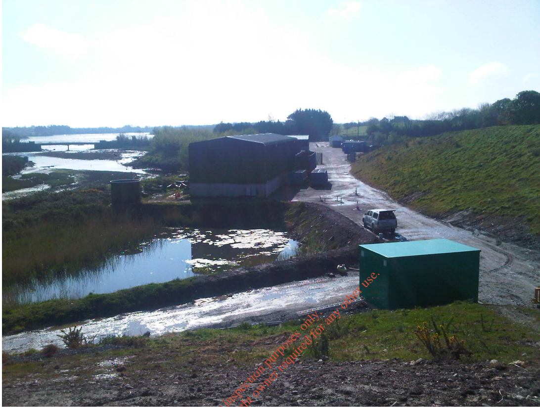
View from pond 5 at the landfill looking down towards the tidal estuary on the left, waste transfer station and civic amenity site, lagoon in forefront and green leachate system control house
