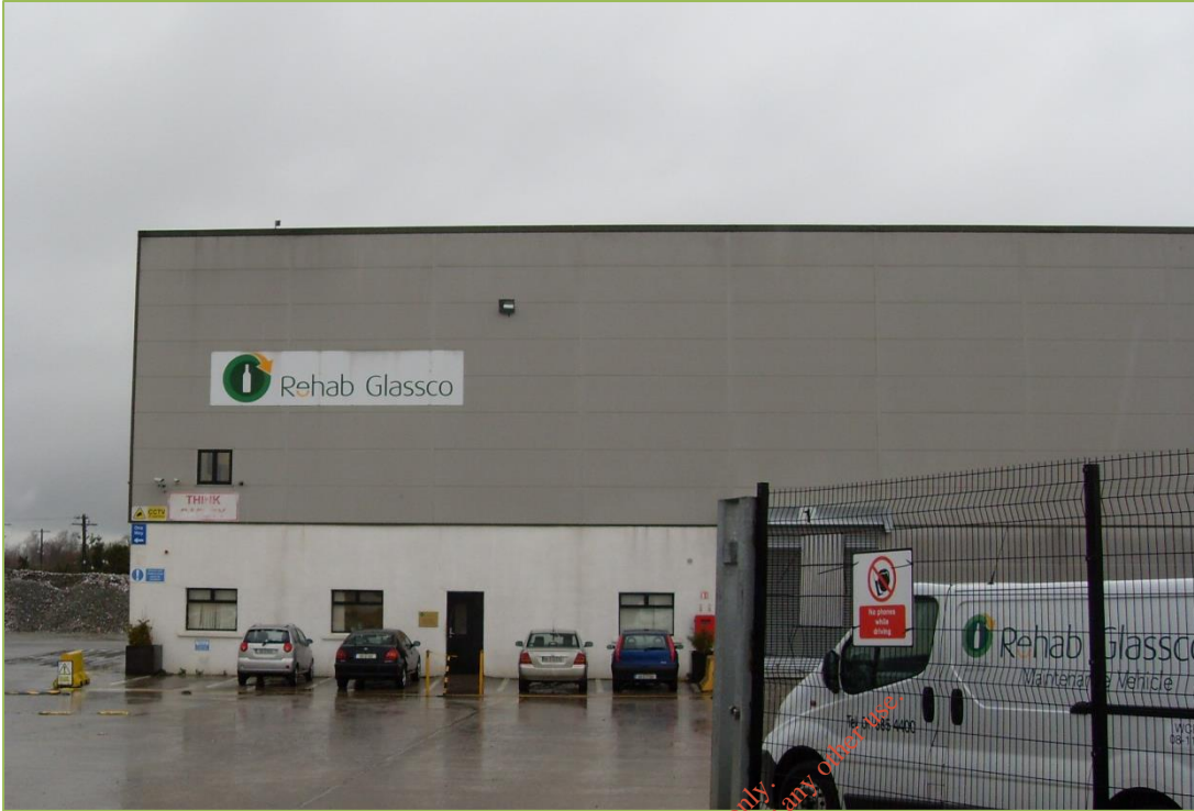
Photograph 1: Main Process Building (including offices)
