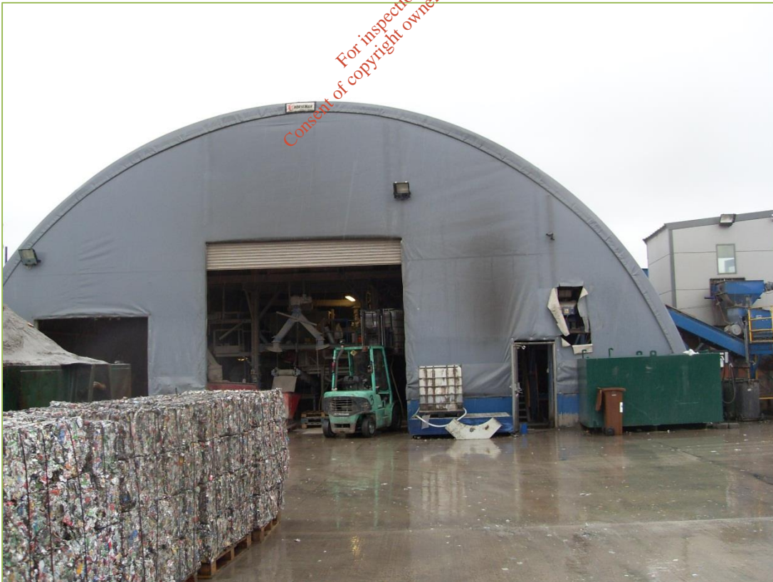
Photograph 2: Drying Plant Building
