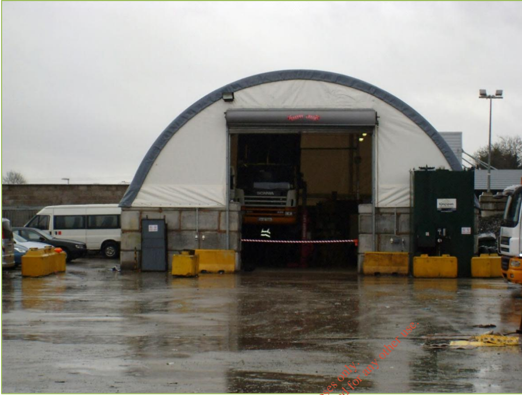
Photograph 3: Vehicle Maintenance Building
