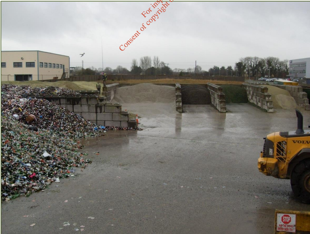
Photograph 4: Input and Output Storage Bays, Concrete Hardstanding
