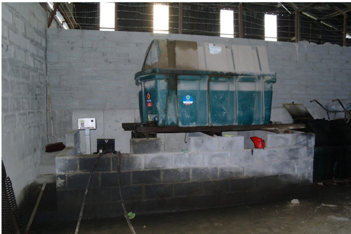
A spill of up to 2,500 litres of gas oil (diesel) in the maintenance shed would be directed to the adjacent yard area. This is an unpaved yard, so we expect a spill of this size to percolate to ground rather than drain to the downgradient site pond, located approximately 200 metres away. The severity of such an event is considered ‘medium’ with clean-up costs between €10,000 and €50,000.
