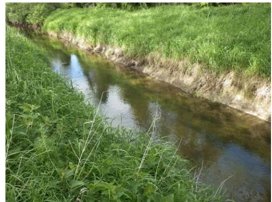
River canalised and dredged
