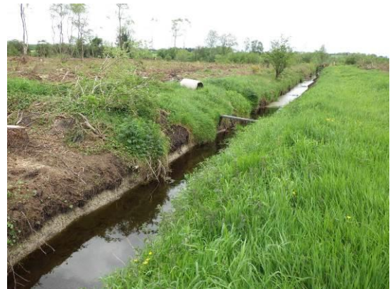
Recently excavated channel
