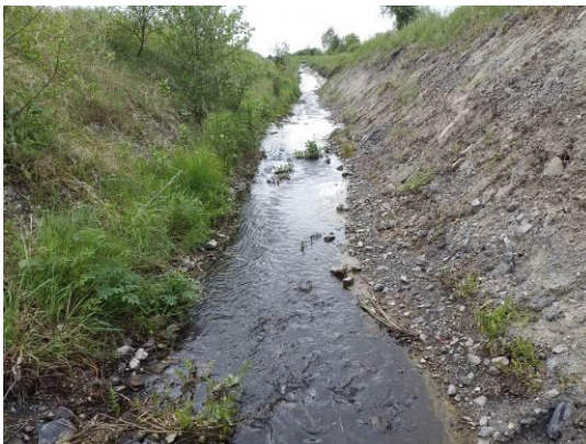
Recently excavated channel on peat with some silty sand and gravel
