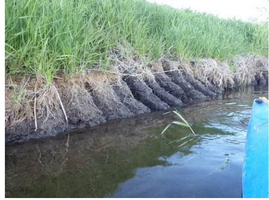
Recently excavated river bank
