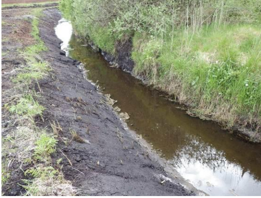
Excavated channel through peat
