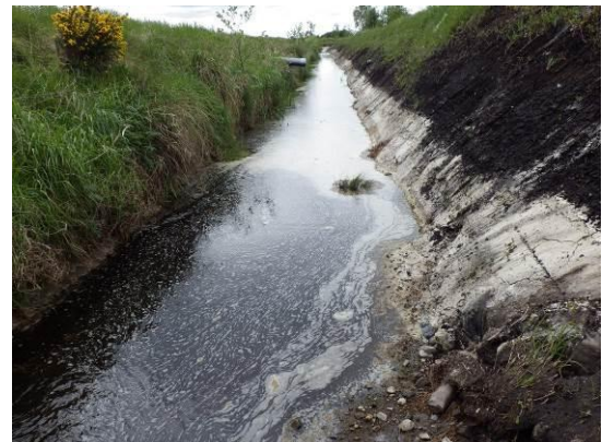
Excavated channel through peat underlain by marl
