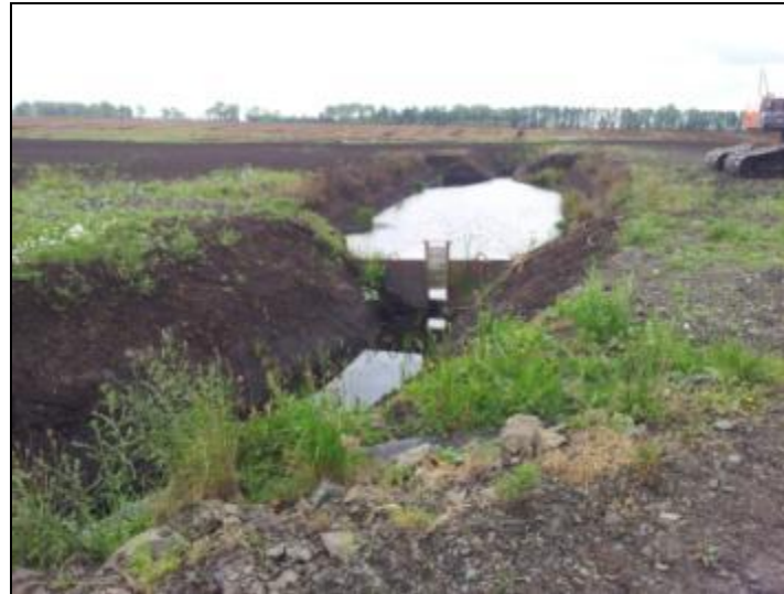
Plate 2.8 Sedimentation basin at Clonsura
