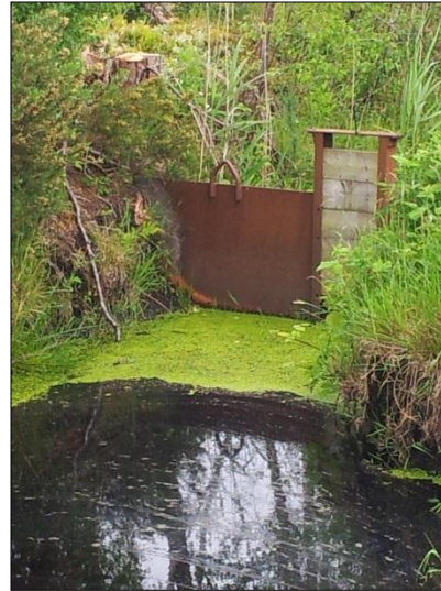
Plate 2.10 Weir located at sedimentation basin at Coole
