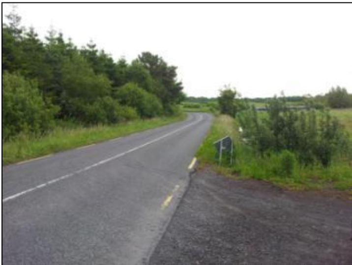
Plate 4.10.1 Main entrance road into Coole site, looking east
